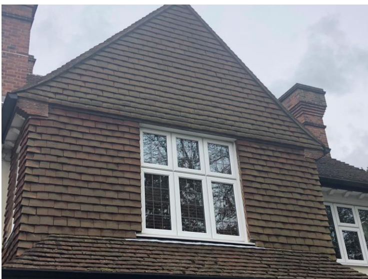
Plate 3. General view of the front cross gable.
