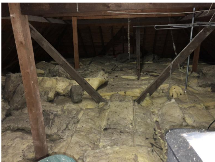
Plate 9. General view of the internal void space of the house.
