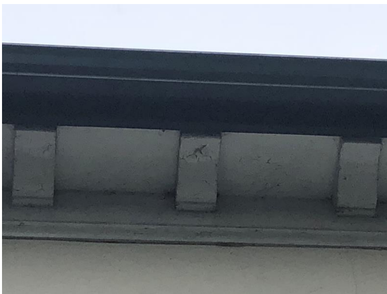
Plate 6. General view of the soffit and fascia.
