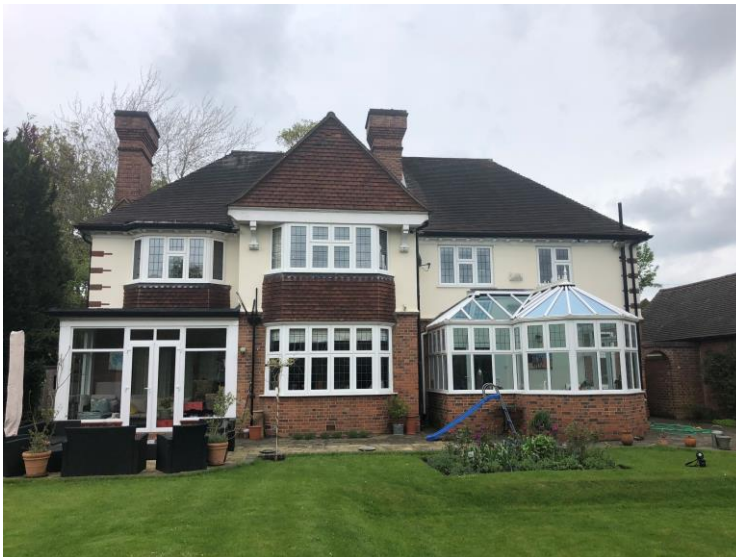
Plate 2. General view of the rear of the property
