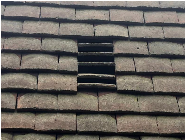
Plate 8. General view of the grilled vents on the garage gable ends.
