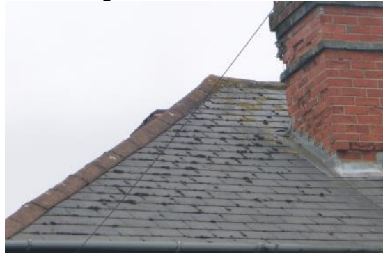
4. Tightly mortared ridge tiles at the front of the house.
