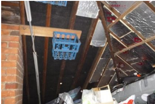
11. Roof partly insulated with bitumen felt and partly with foil covered insulation panels.
