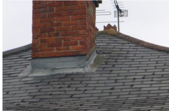
10. Tight lead flashing around chimney at rear of the house.
