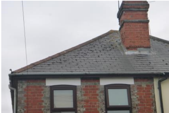
3. Tightly fitted, flat slate roof tiles.
