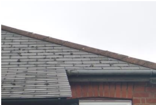
5. Tight hip tiles at the rear of the house.
