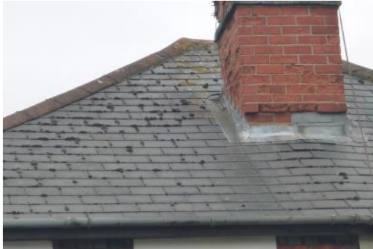
9. Tight lead flashing around chimney at front of the house.
