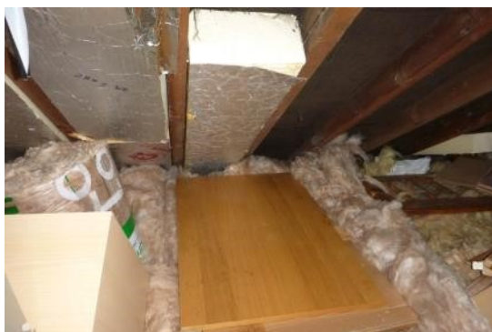
13. Fibreglass insulation extending to eaves in some places.
