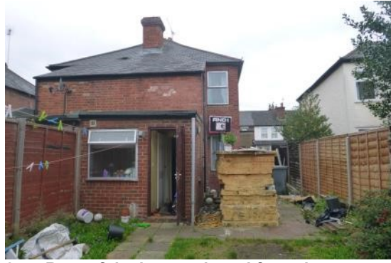
2. Rear of the house viewed from the west showing the flat-roofed extension.
