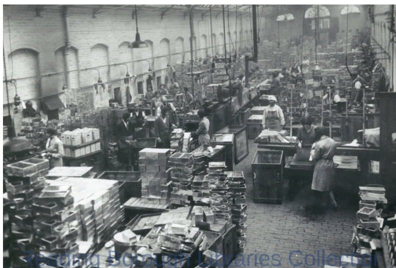
Plate 10: Interior of the Tinplate Factory of Huntley, Boorne and Stevens, at London Street, Reading, c. 1930
