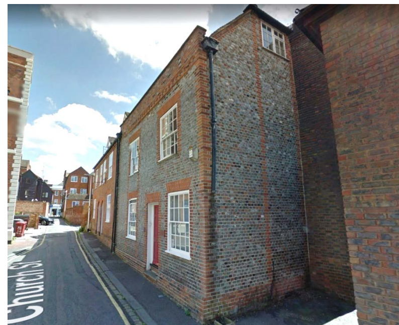
Plate 21: No. 11 Church Street.
