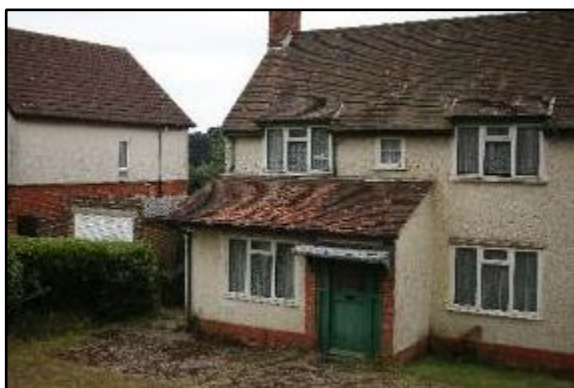
Photo 51: building 203 north elevation
