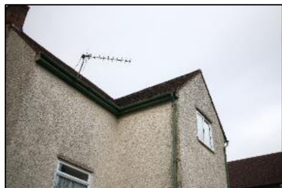
Photo 52: building 203 southern elevation
