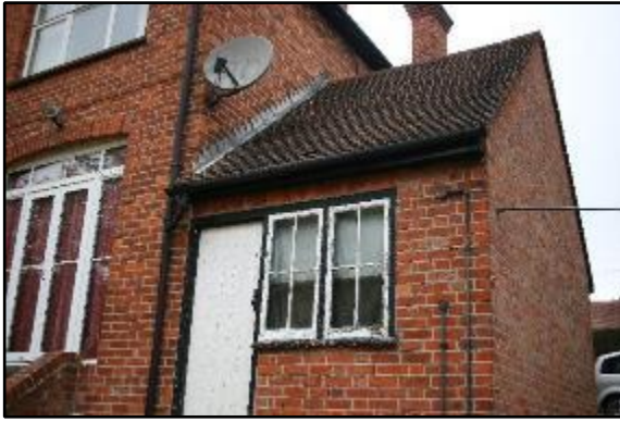
Photo 32: building 199 rear porch (east)
