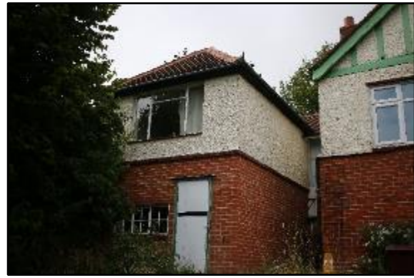
Photo 44: Building 201 south elevation
