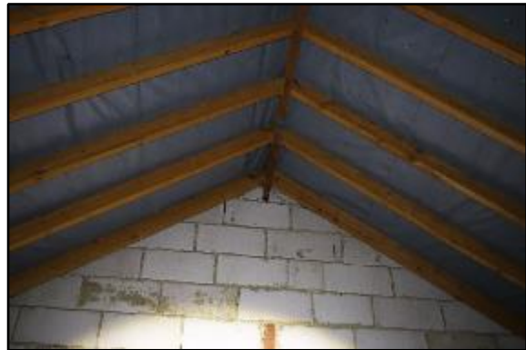
Photo 37: building 199 new loft
