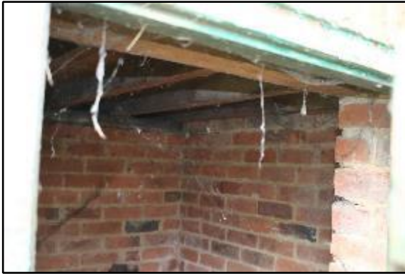
Photo 53: building 203 coal shed
