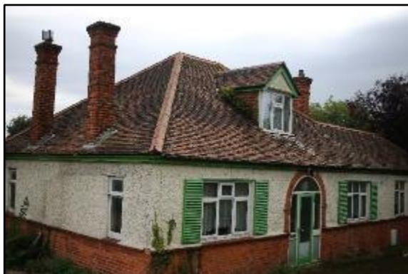
Photo 41: Building 201 – northern elevation
