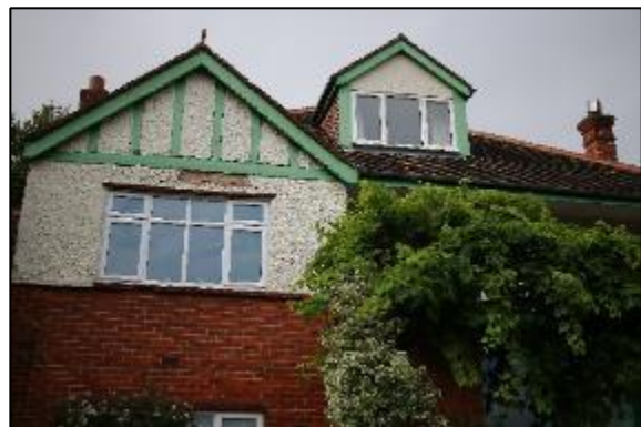
Photo 42: Building 201 – south elevation
