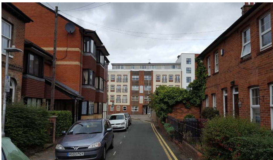
View from Newark Street looking north to Crown Street frontage
