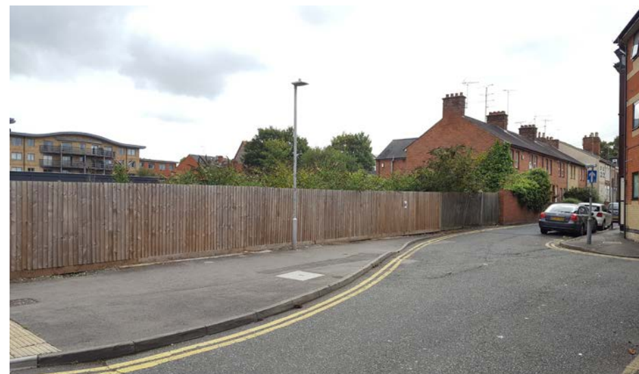
View of west side of application site with Newark Street terrace to right. Note; tapering and termination of pavement on application site side of road
