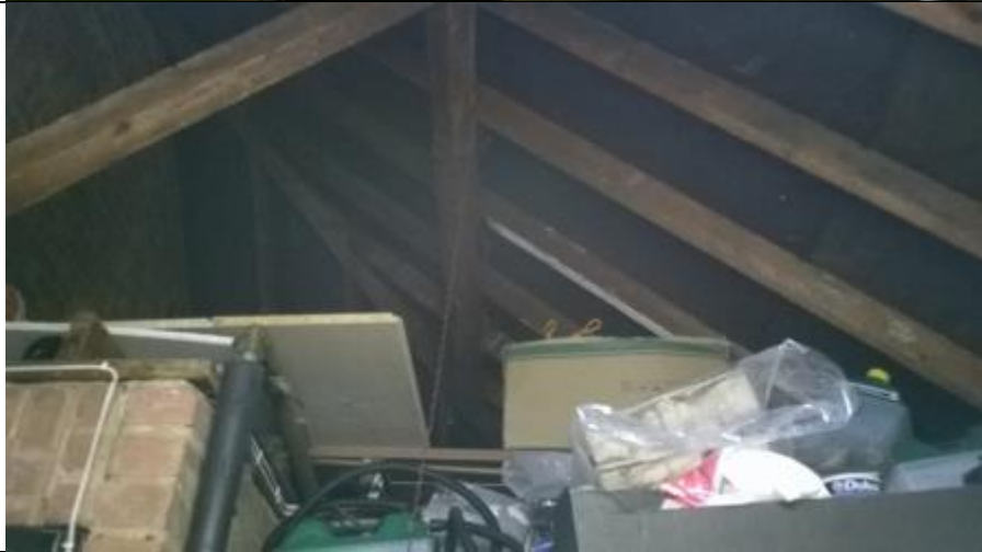
Photo 2: internal garage roof structure.
