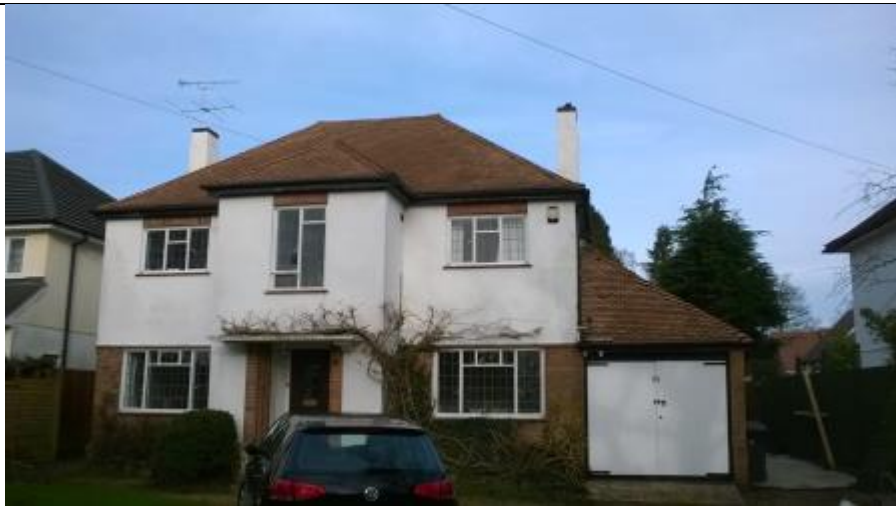
Photo 1: front of the building.
