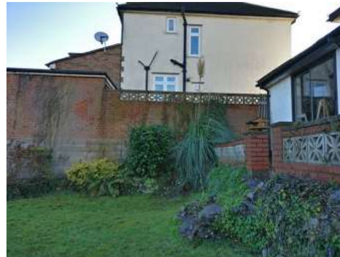
No. 330 side extension wall considered overbearing
