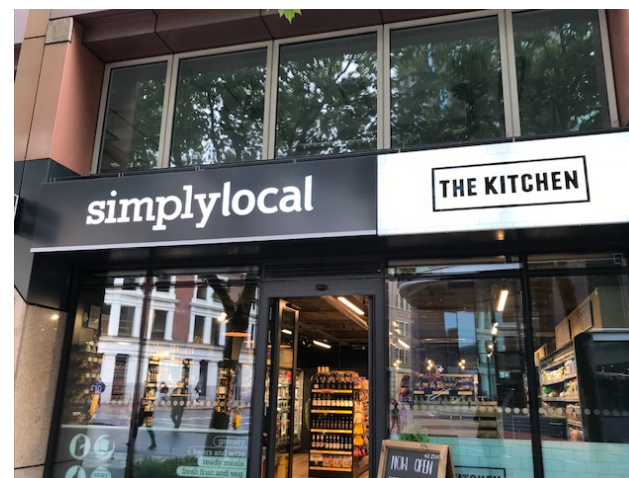
Simply Local: Use of internally illuminated façade panel to front elevation
