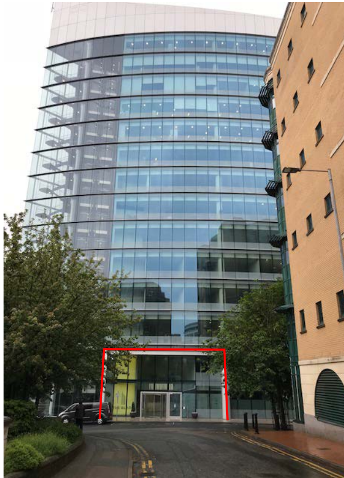
Existing View of The Blade Front Elevation
