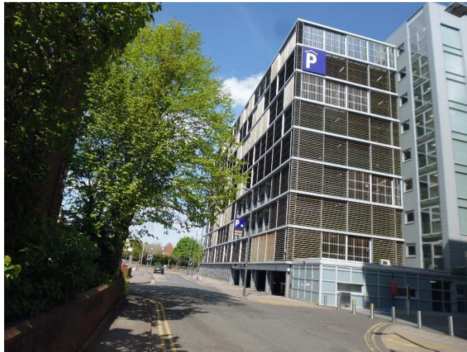
Photo 11: Q-Park Chatham Place Multi-Storey Car Park
