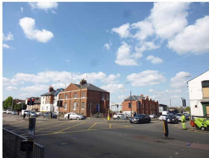
Photo 1: Oxford Road/Bedford Road Signalised Junction
