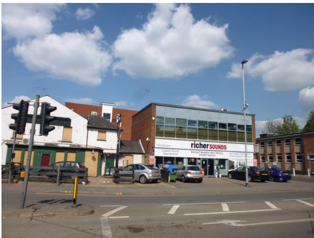
Figure 50, 51, 52 – The existing landscaping of the application site:
