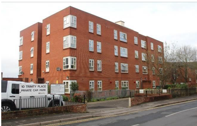
Figure 15, 16, 17 - Sheltered housing at 10 Trinity Place Top – from the south west and showing the relationship to the two buildings on the application site Middle – West elevation facing Bedford Road Bottom – East elevation facing Trinity Place
