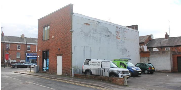
Figure 7, 8, 9, 10 – The Richer Sounds store at 118 Oxford Road: ( Top left ) – Front elevation (south) to Oxford Road ( Upper left ) Side elevation (west) to Bedford Road ( Top right ) Side elevation (east) to Trinity Place ( Bottom right ) Rear (north) elevation
