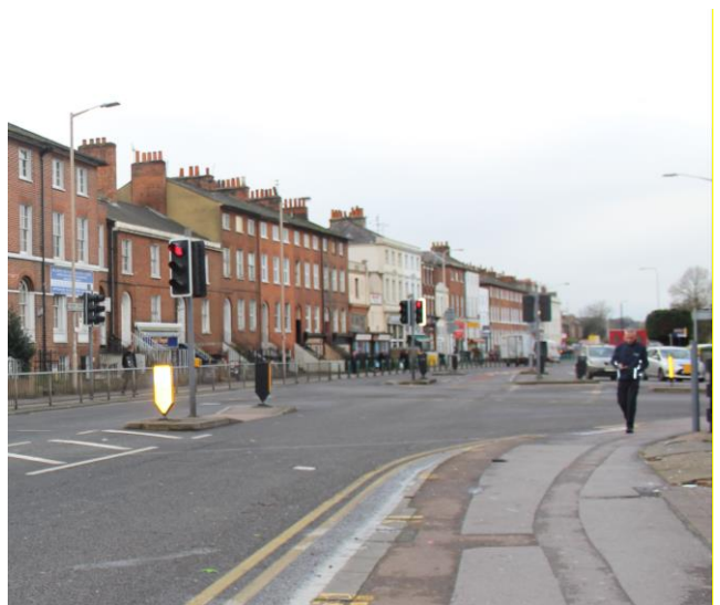
Figure 62, 63 + 64 The existing context at the corner: (Top) The existing licensed premises at the north east side of the junction. (Middle) 120 Oxford Road presents a more or less blank flank wall to the west side of the junction. (Bottom) Terraced housing on the south side of the junction.
