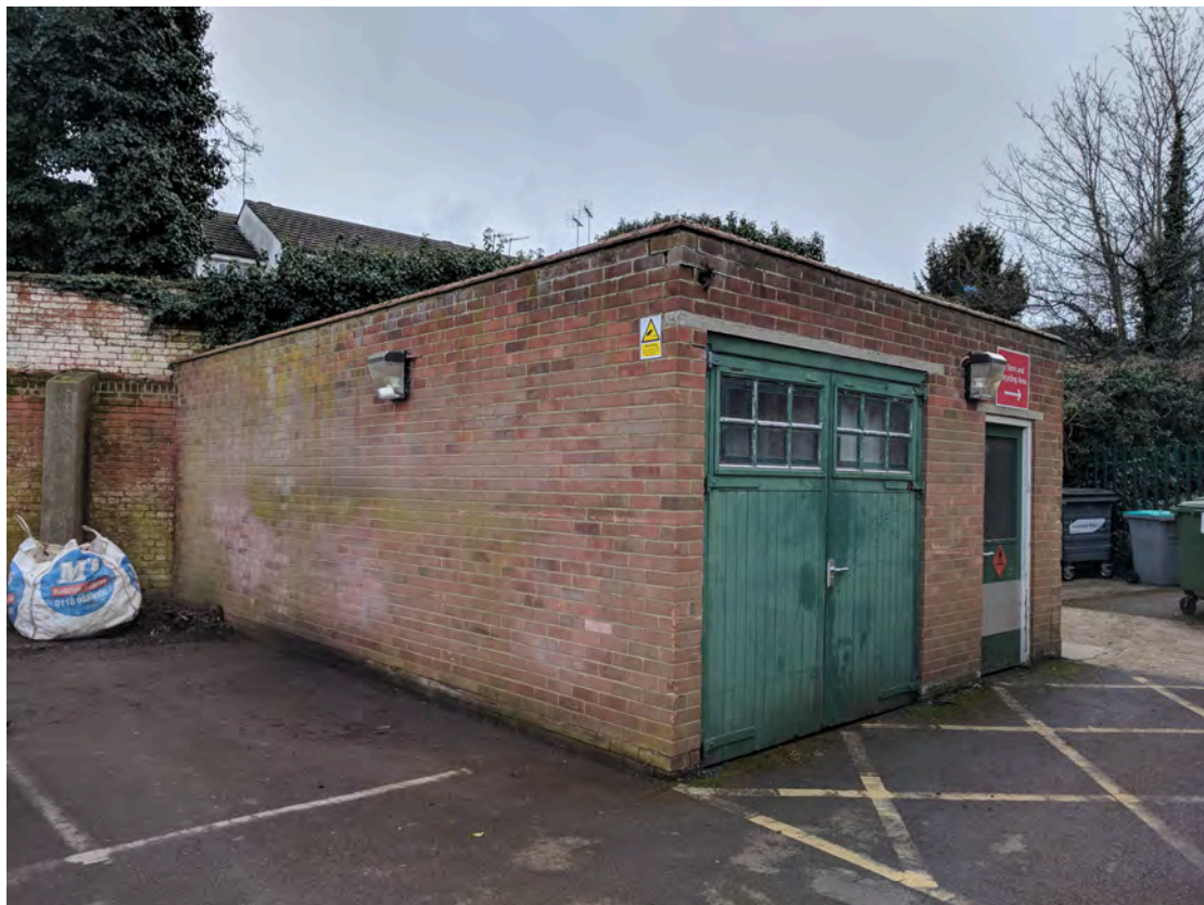
Fig.1: Front view of garage
