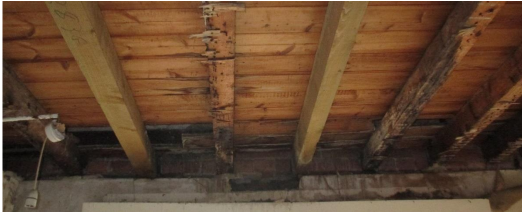
Figure 5.63 - Exposed ceiling joists in the southern room show that some of this structure has been replaced with modern timbers
