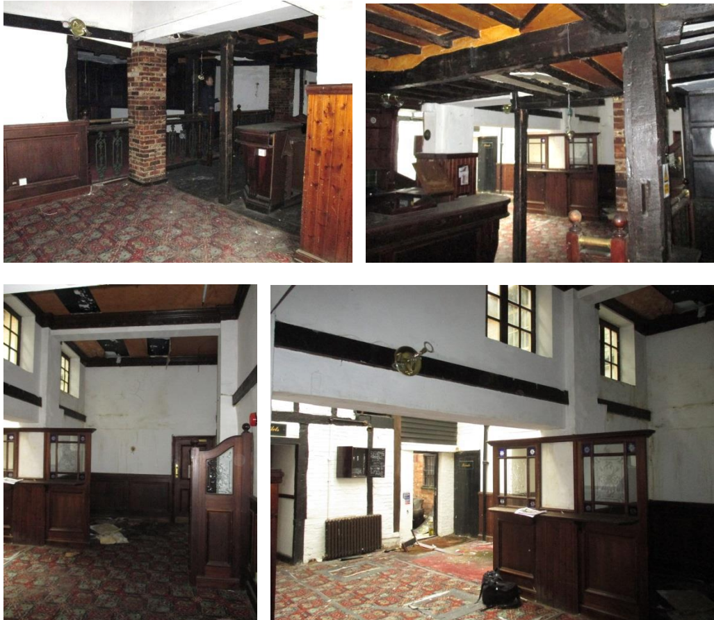
Figure 5.46 – Some demolition of the historic rear elevation has occurred to open up the space to the modern rear extensions
