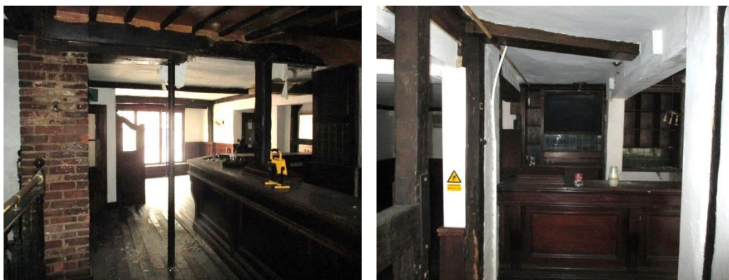
Figure 5.42 – The modern bar in the centre of the floor plan compromises the plan form of the northern premises (L) and central passageway (R)
