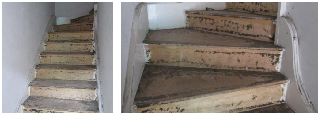
Figure 5.50 – Staircase at the front of the building, accessed via a separate entrance
