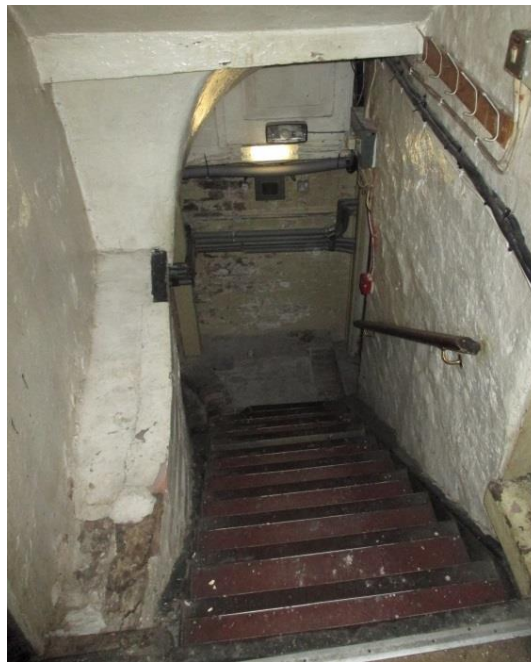
Figure 5.32 – Staircase to basement level
