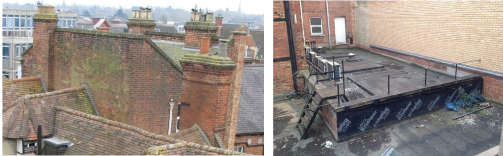
Figure 5.78 – Roof forms at No.32 Market Place
