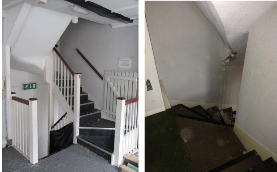
Figure 5.14 – A single, narrow staircase runs throughout the building
