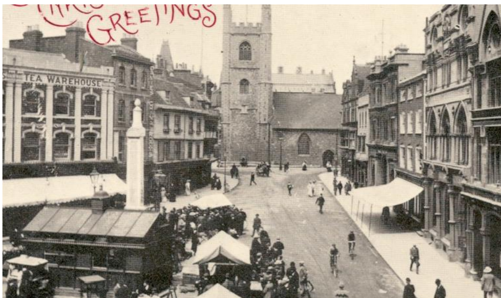
Figure 5.22 –No.27 and 28 form part of the commercial building stock on the Market Place, where the key commercial activity in Reading was concentrated
