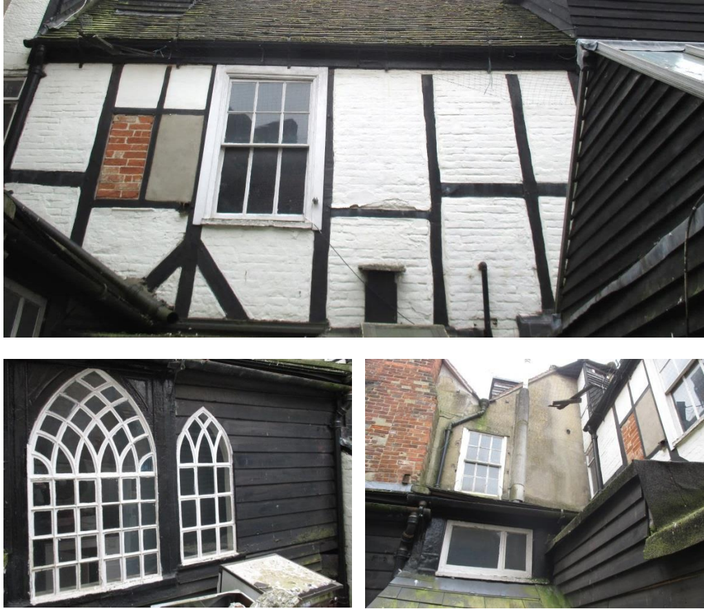
Figure 5.27 – Areas of exposed timber-framing, weatherboarding and cement render
