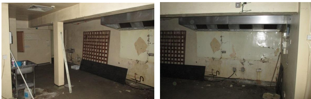
Figure 5.48 – Former kitchen area in the modern rear extension at ground floor
