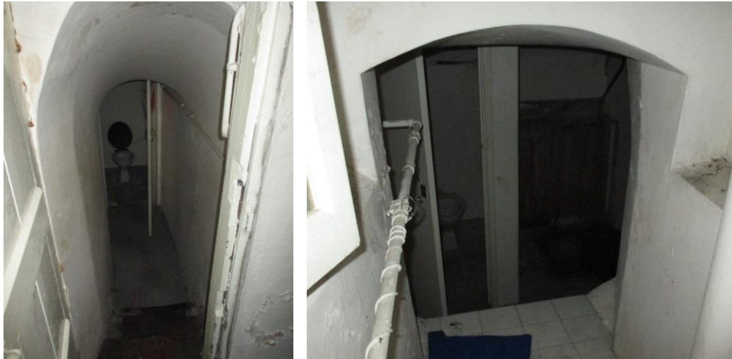
Figure 5.16 – Vault space under the street at basement level reflects the building's historic use as commercial premises
