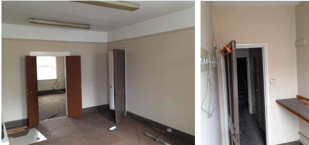
Figure 5.85 – The historic layout of two principal rooms, with two additional smaller spaces survives at second floor level
