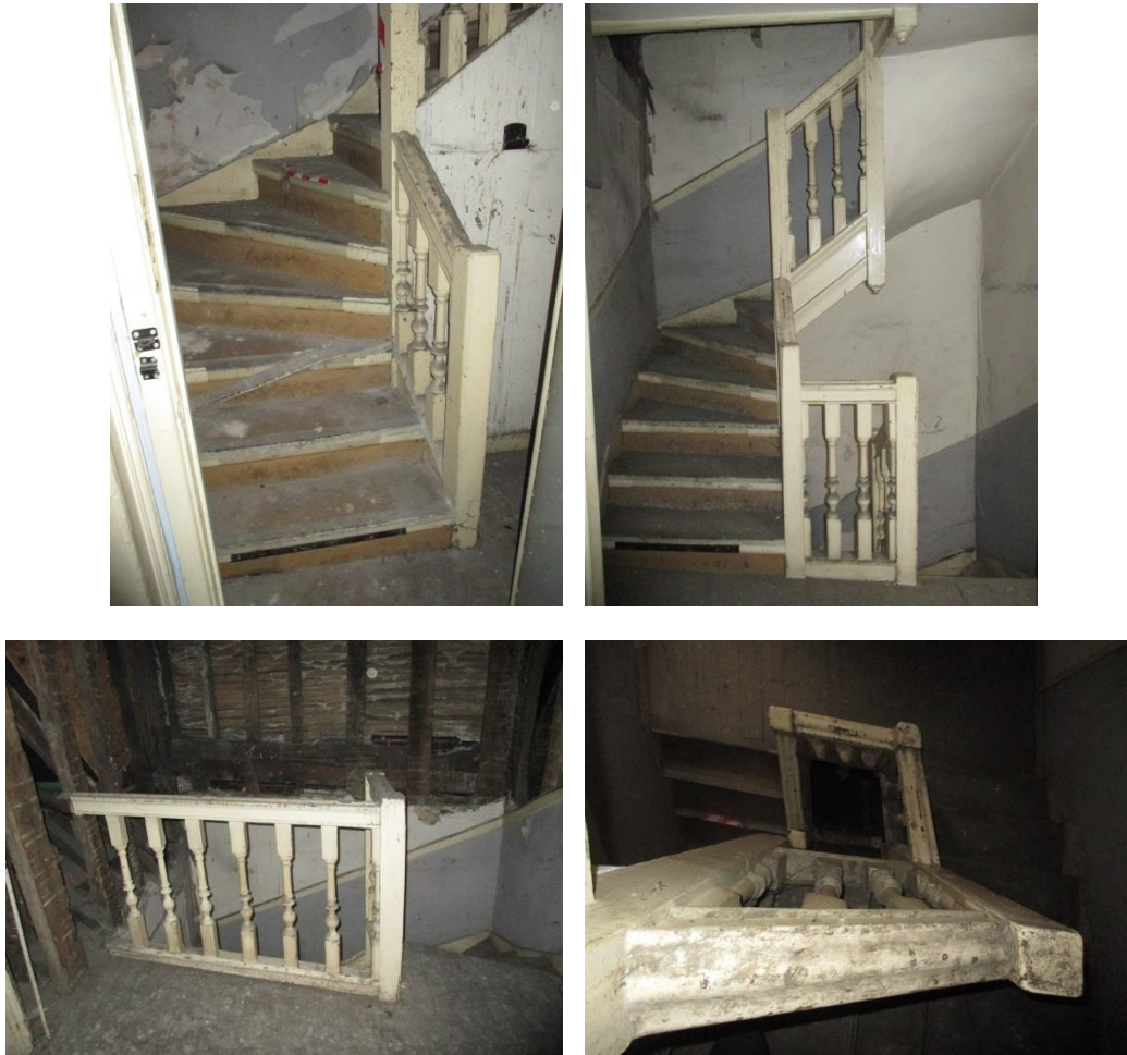
Figure 5.60 – The framed newel stair is typical of 17 th century style, and extends between the first and third floor levels of the building
