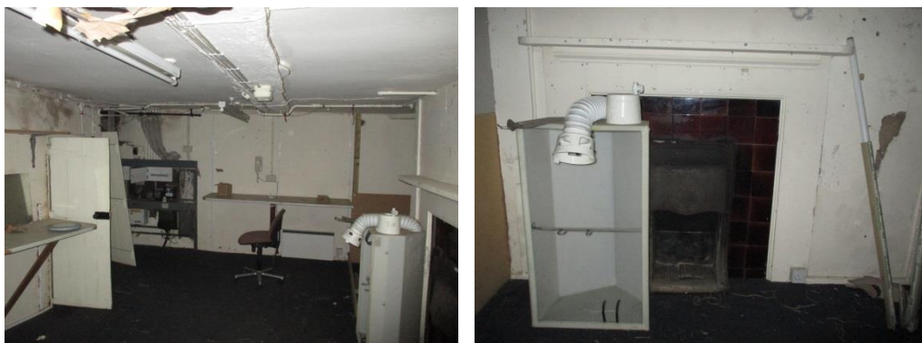
Figure 5.15 – Timber beam and fireplace at basement level
