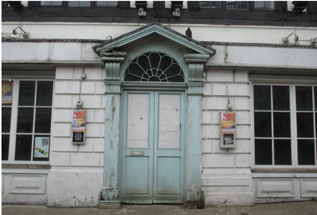
Figure 5.29 – The central doorcase windows are products of the late-20 th century
