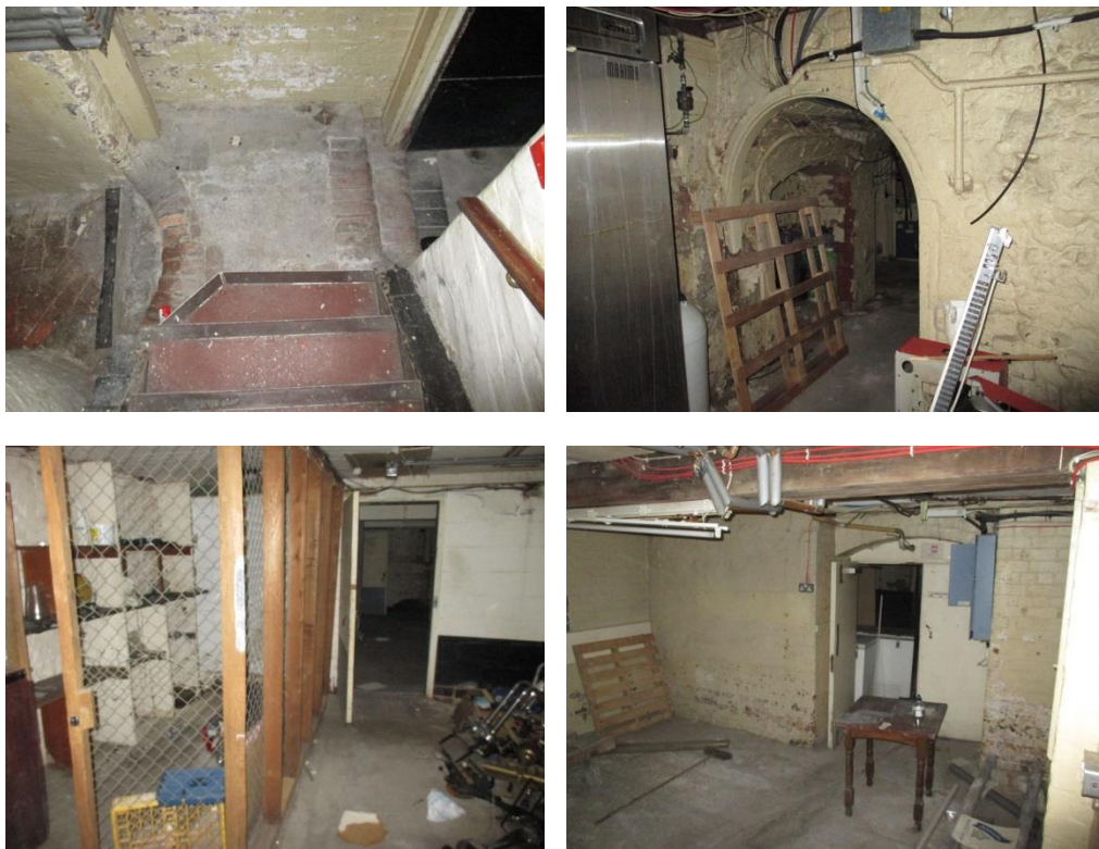
Figure 5.34 – Four rooms under the historic portion of the building are connected by passageways at the front and back of the house
