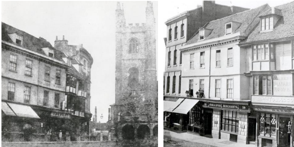
Figure 5.24 – Photographs of 1845 and 1860, showing The Coopers public house with plain render to the street elevation
