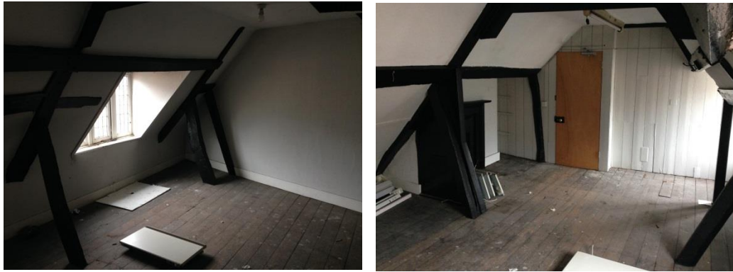
Figure 5.21 – The rafters and purlins of the roof structure are exposed at the third floor
