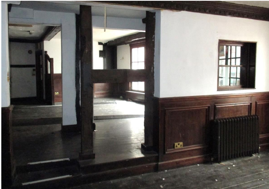
Figure 5.41 – Lateral openings in the spine walls have compromised the legibility of the two separate premises with a central passageway
