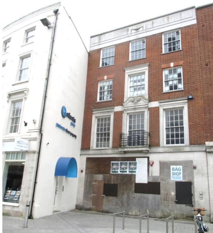
Figure 4.27 – No.175 Friar Street
