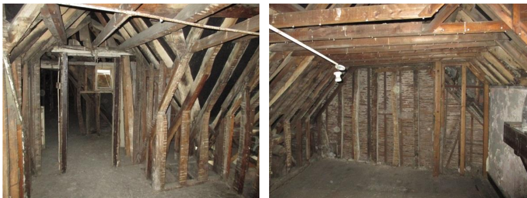
Figure 5.70 – At third floor level the structural timbers are completely exposed, and comprise original 17 th century beams as well as areas of replacement
