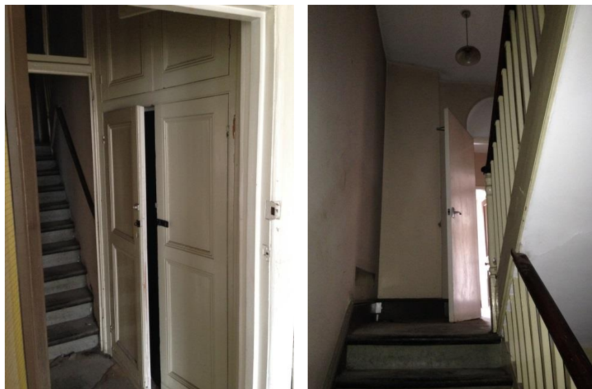
Figure 5.84 – The staircase between first and third floor level is original
