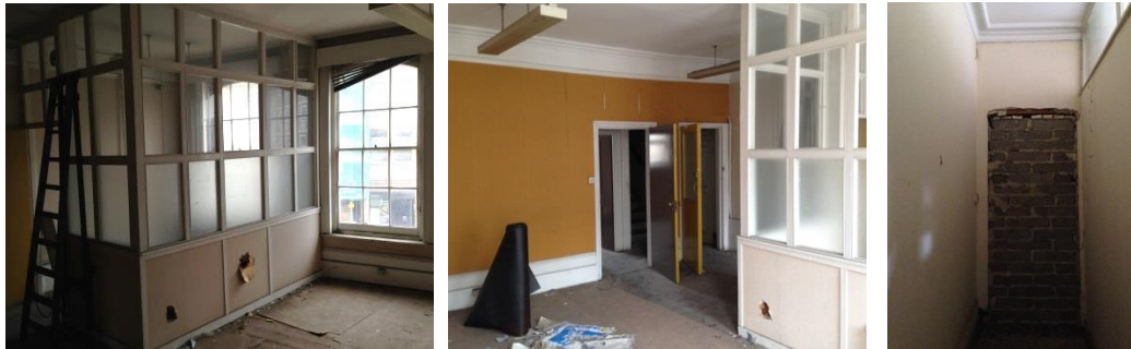
Figure 5.82 – Modern partitioning has compromised the traditional two-room floor plan
