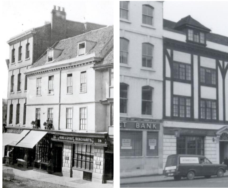
Figure 5.76 – The front elevation remains largely intact, with some slight alterations
