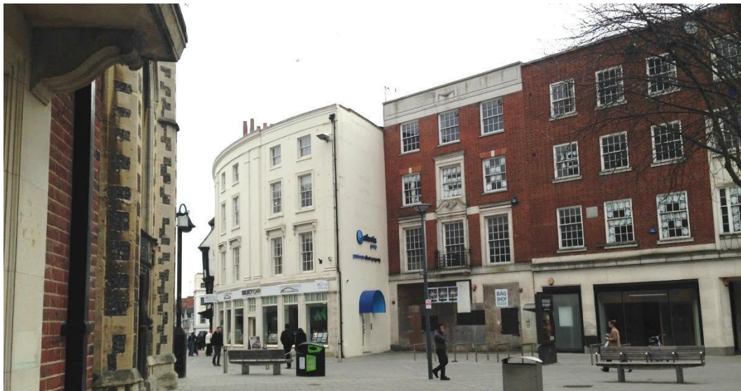
Figure 4.19 – The reconstruction at Nos.173-175 Friar Street has created an awkward kick-out in the previously smooth, curved building line
