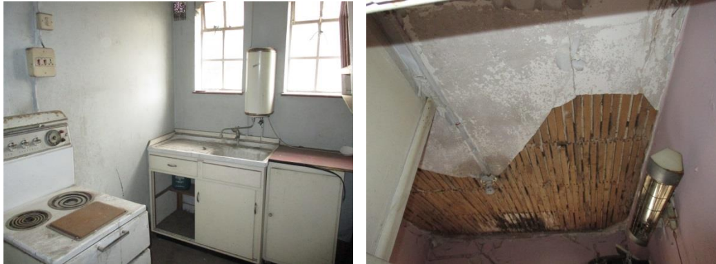
Figure 5.68 – Bath and utility rooms in the modern extension
