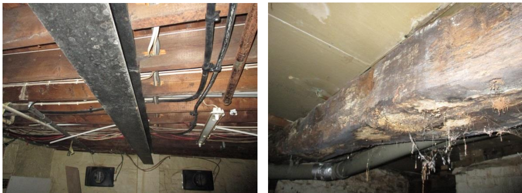
Figure 5.36 – Historic and more recent timbers at ceiling level
