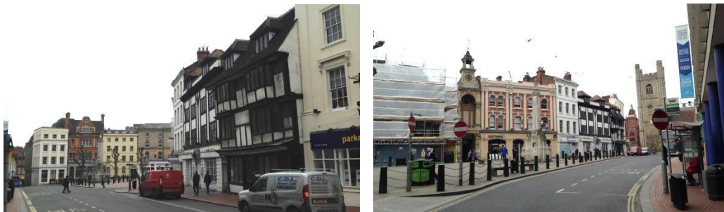
Figure 5.72 – No.32 is listed for group value, and it forms a part of the historic building group around the Market Place
