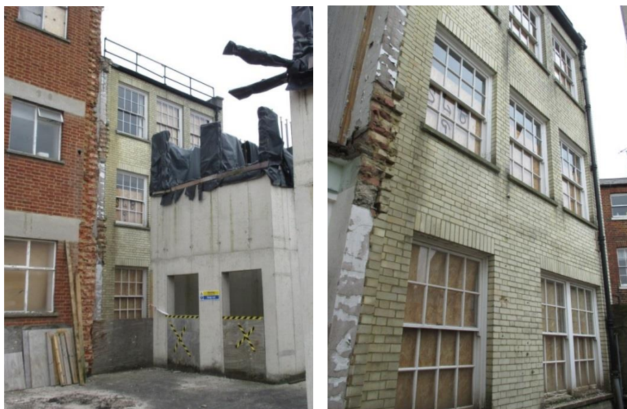
Figure 4.28 – The rear elevation is not visible from the public realm
