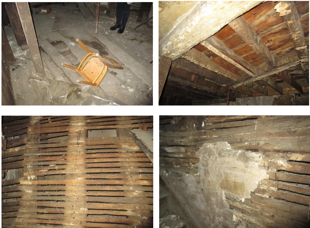
Figure 5.57 - Large parts of the structure in this 17 th century room are original
