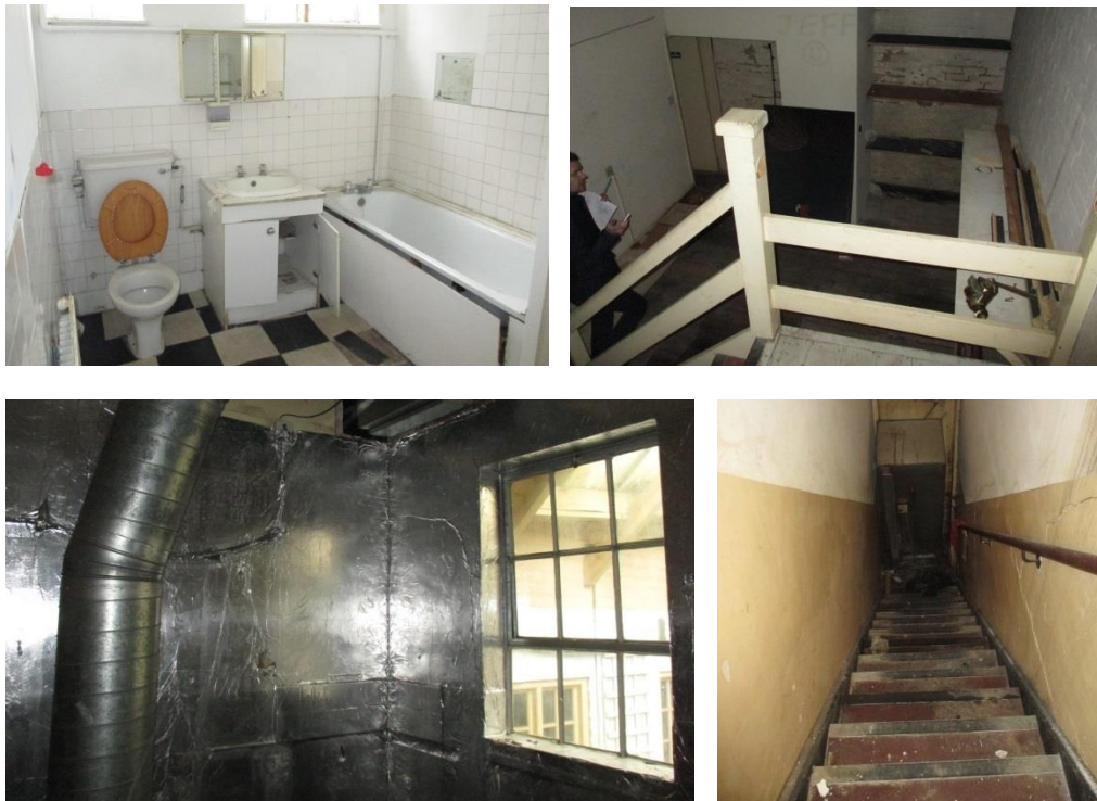
Figure 5.59 – The ancillary rooms within the 20 th century extensions
