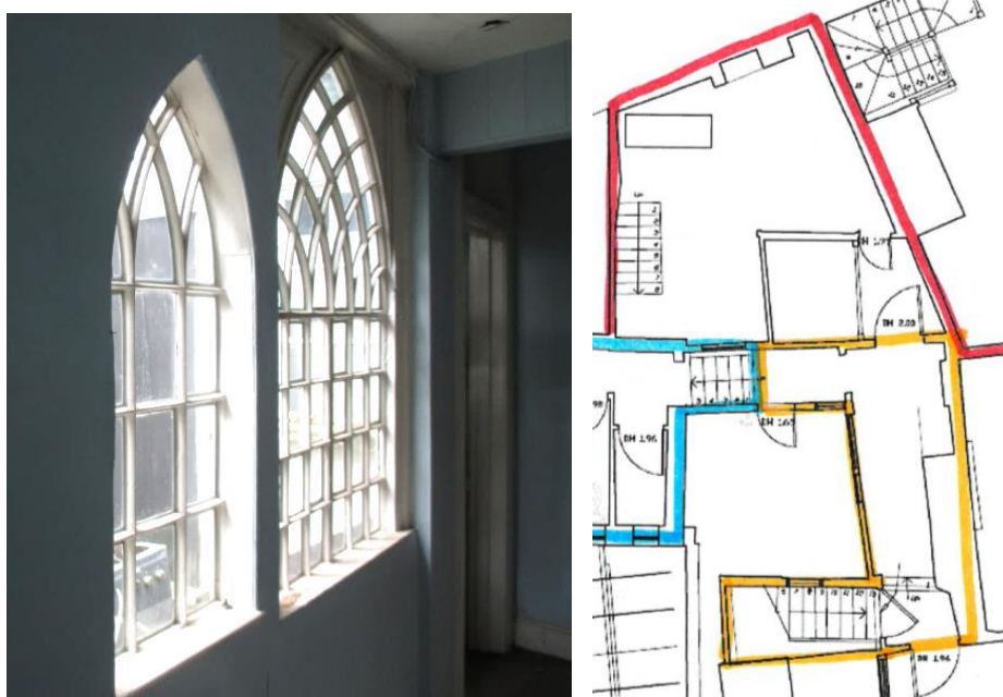
Figure 5.55 – A corridor was added in the early-19 th century to the back of the 17 th century range fronting the street, to provide access to the newly-acquired room
