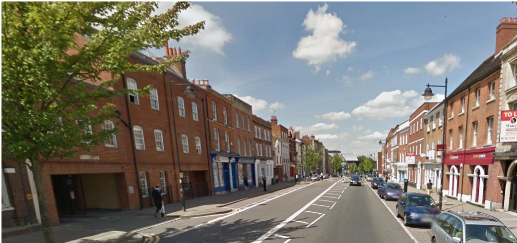
Figure 4.9 – London Street is a broad, strongly linear route, with a high number of surviving historic buildings
