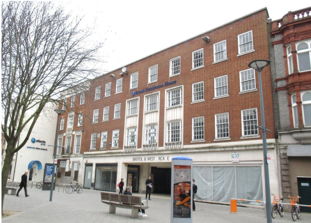
Figure 4.21 - No.173-175 Friar Street present an unkempt and run-down appearance, directly overlooking the key space of the Town Hall Square
