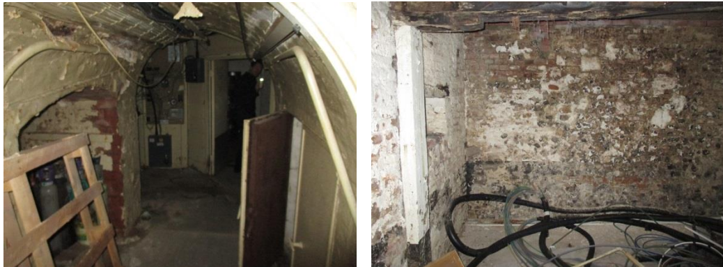
Figure 5.35 – Street alcoves and some wall fabric indicate the incorporation of an older building at basement level
