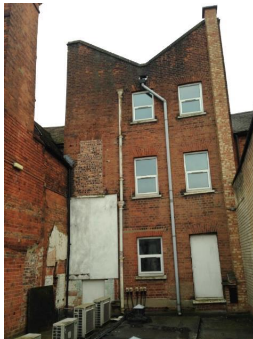
Figure 5.77 – Rear elevation of No.32 Market Place
