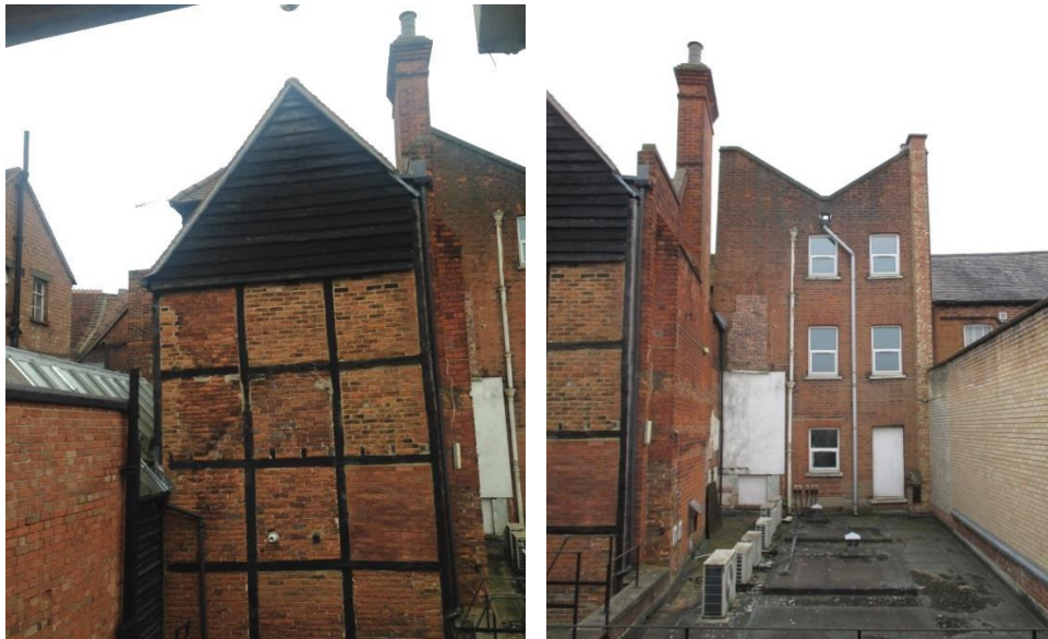
Figure 5.31 – The long rear range has exposed timber-framing, and a brick retaining wall where the original third bay was demolished between 1842 and 1860
