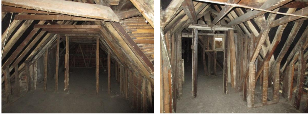
Figure 5.31 – The roof structure of the 17 th century core is exposed at attic level, and appears to be relatively intact
