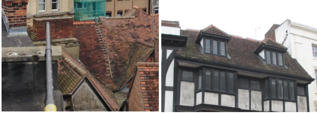
Figure 5.12 – The roof of Nos.27 and 28 Market Place
