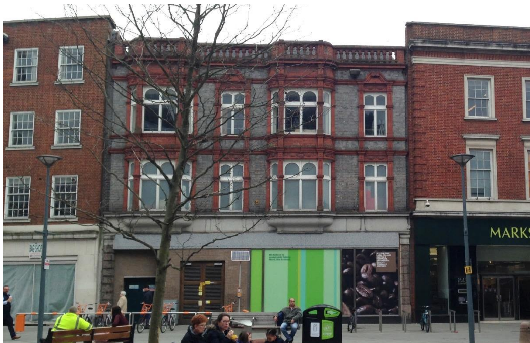
Figure 4.23 – No.172 Friar Street formed part of the same development as Nos.173 and 174 Friar Street, and was built to the same design
