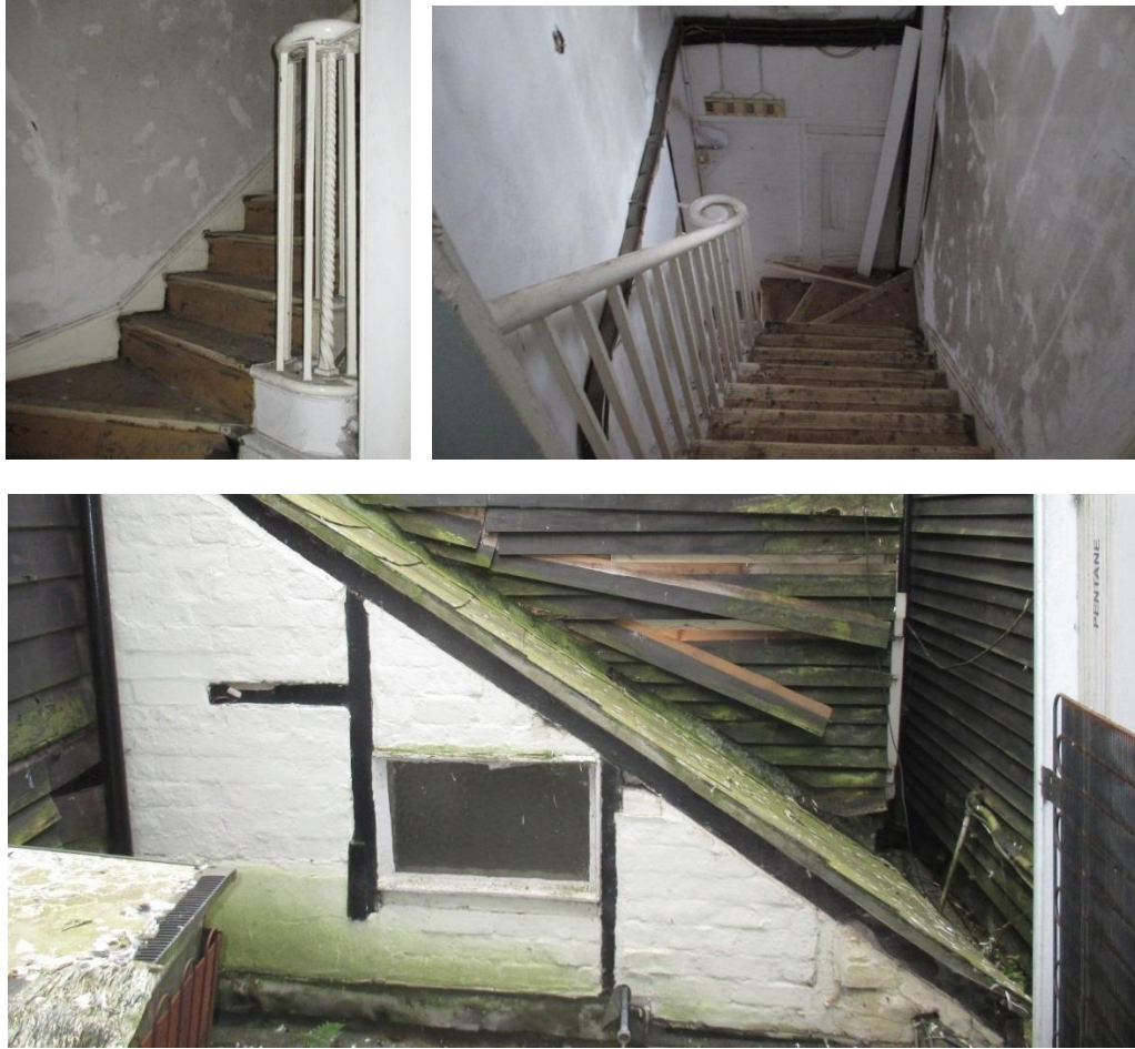
Figure 5.54 – Staircase in the centre of the building
