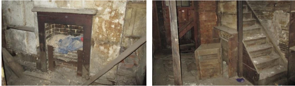
Figure 5.58 – The 17 th century northern room incorporates a fireplace and stair
