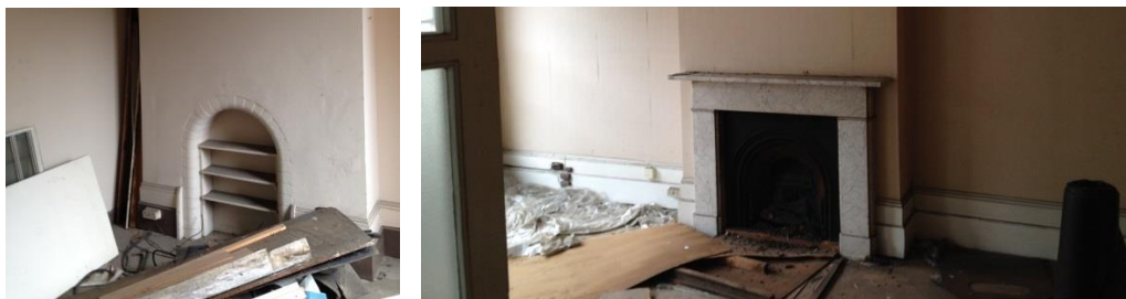
Figure 5.83 - Some original decorative fabric and features survive, including the fireplaces in each room
