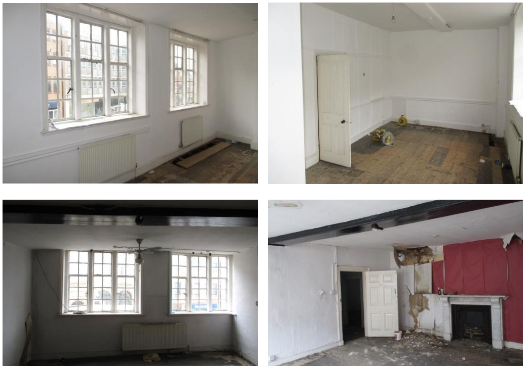
Figure 5.51 – Two rooms to the front of the building retain their original proportions
