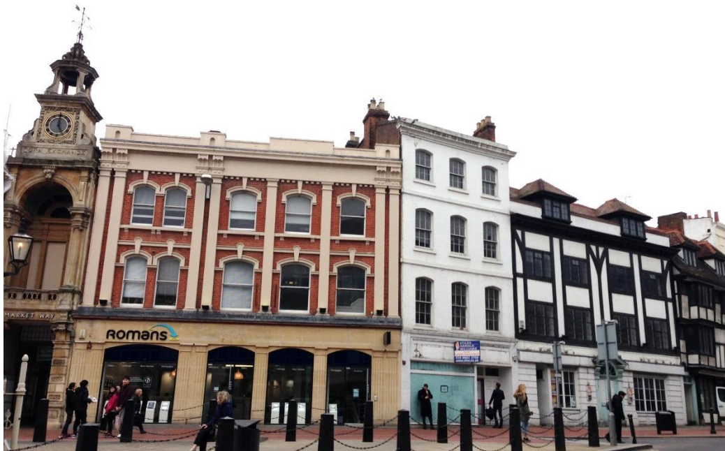
Figure 6.12 – The former bank forms part of a building group composed of historic, listed buildings in a mixture of commercial uses
