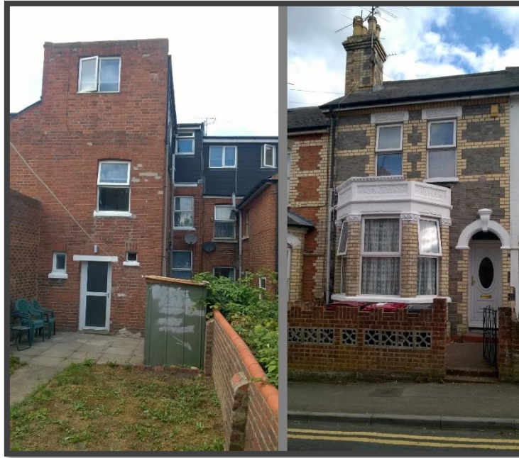
3. External appearance to be retained.
