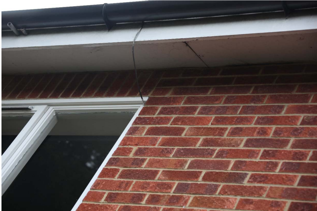
Fig. 5 – South Facing Eaves
