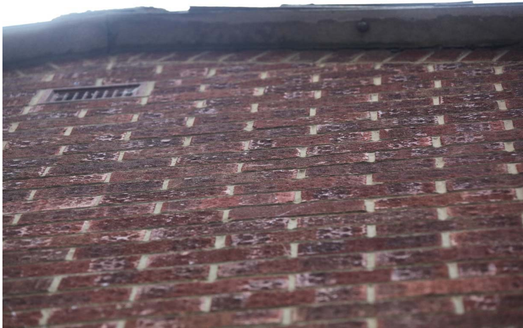
Fig. 3 – East Facing Gable Verge
