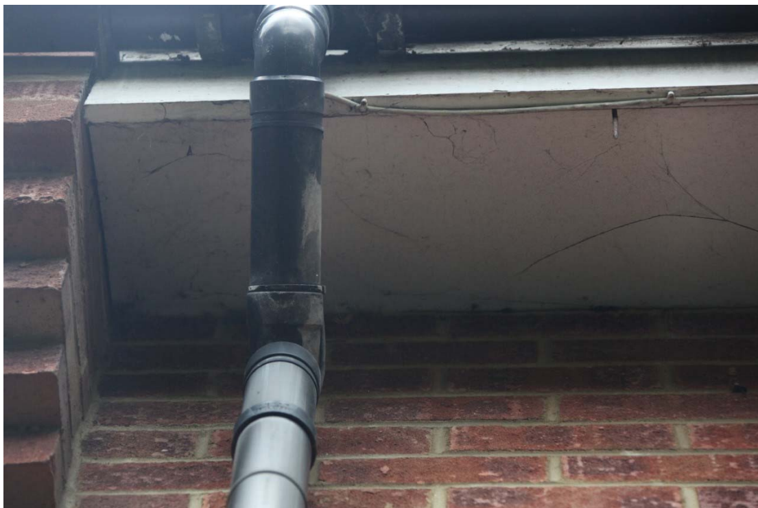
Fig. 6 – South Facing Eaves
