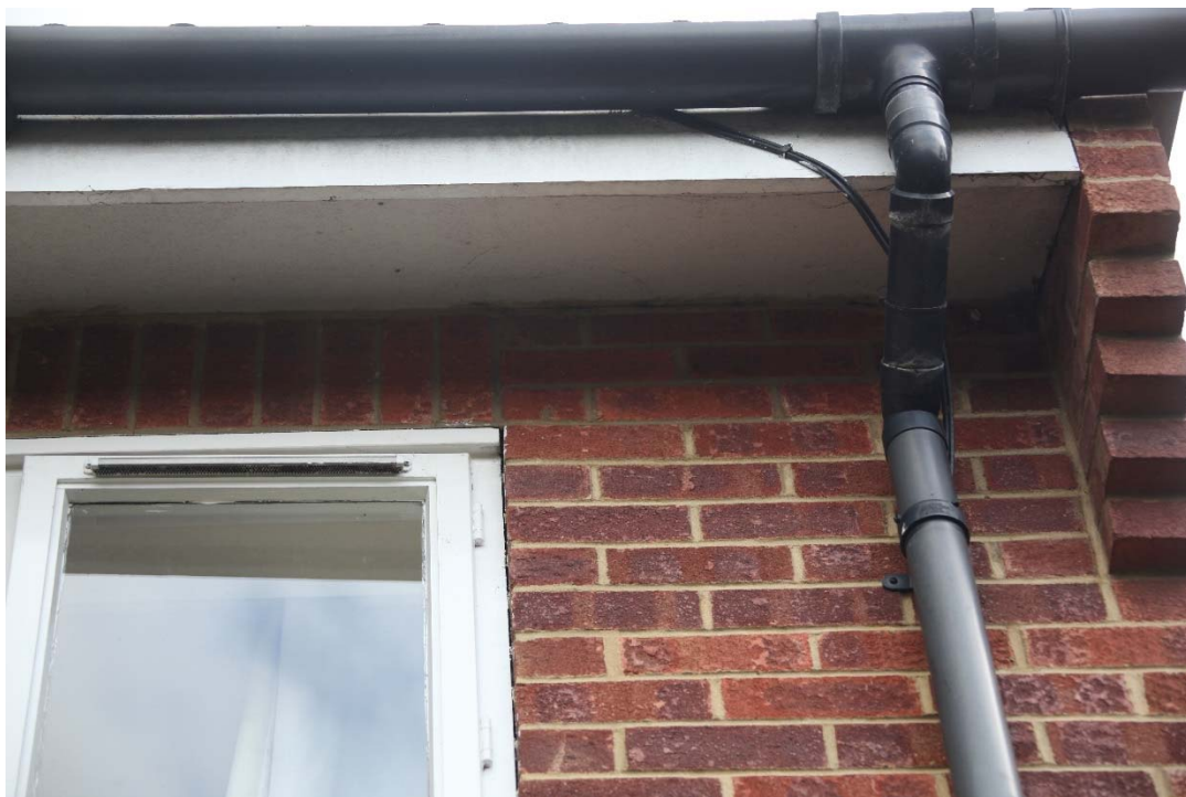
Fig. 4 – North Facing Eaves
