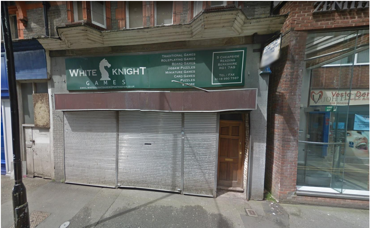
The View of the east façade (Front) of the property
