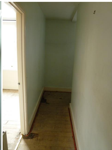
Stud wall to be removed
