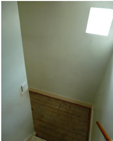
New stud wall to be position at the bottom of the stairs
