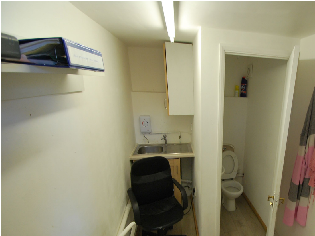
Toilet area - to be improved but retained
