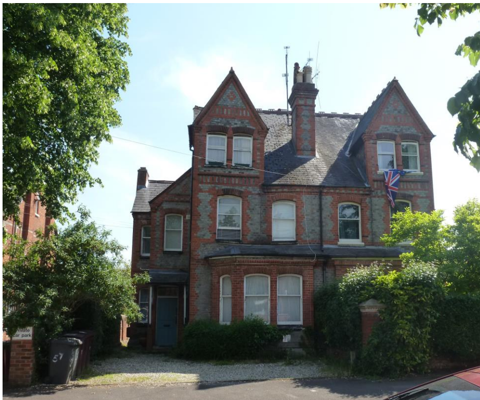
Fig.1: View of 57 Alexandra Road from the street
