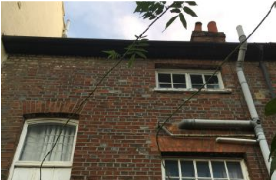
Figure 1 Drainage pipes from existing shower room
