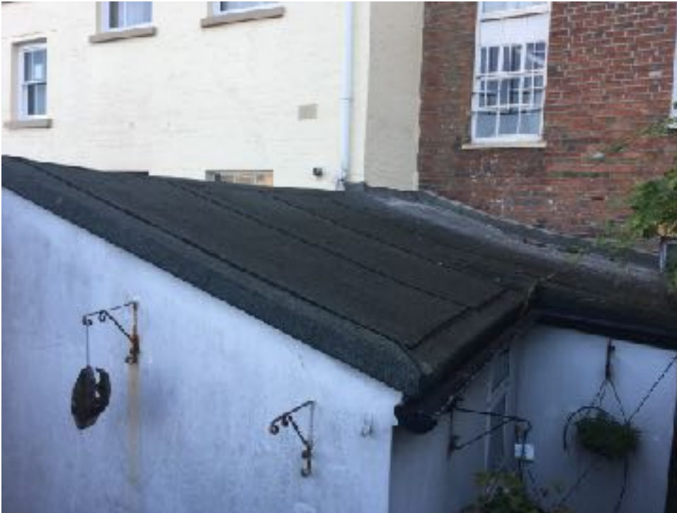
Figure 2 Flat roof over rear extension
