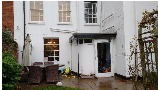
1970's wc extension
