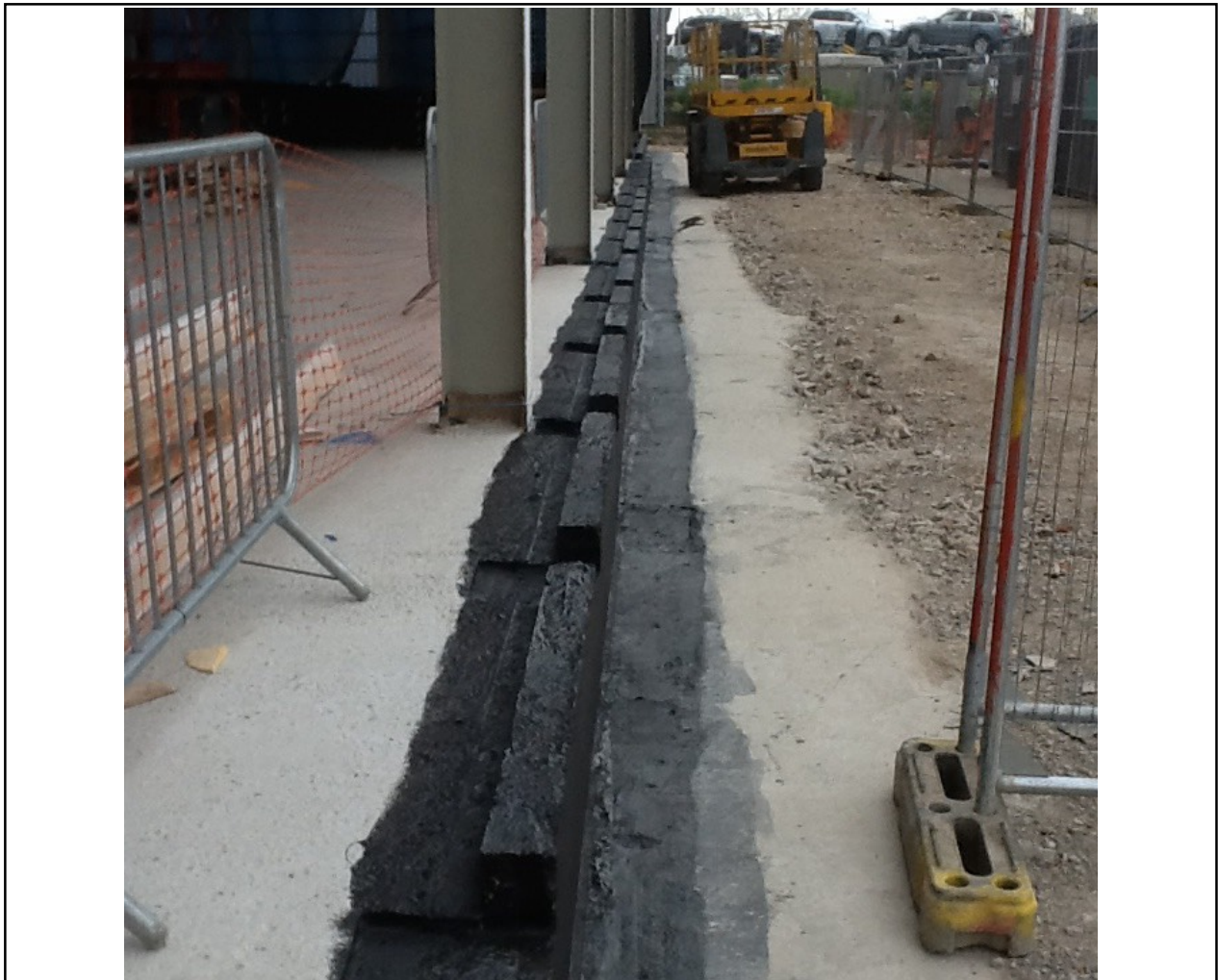
Wall 1 , viewed from corner of intersection with wall A
