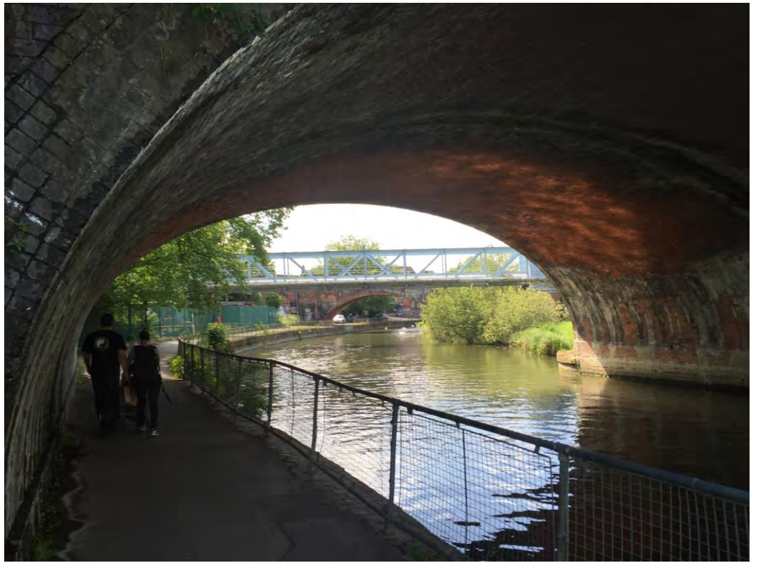
Plate 4 Looking south from under listed bridge towards non-designated historic bridge
