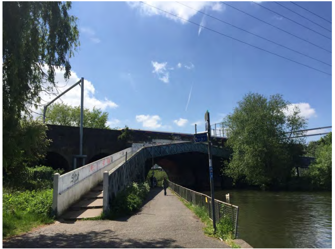
Plate 2 Looking south towards listed bridge
