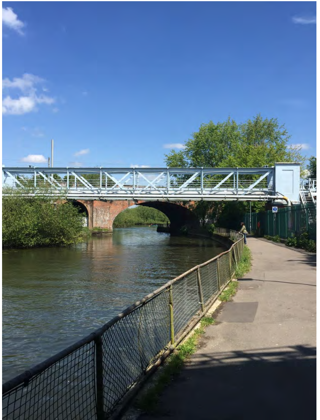
Plate 1 Looking north towards listed bridge
