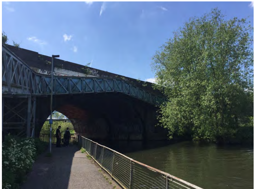
Plate 3 Looking south towards listed bridge (close up)
