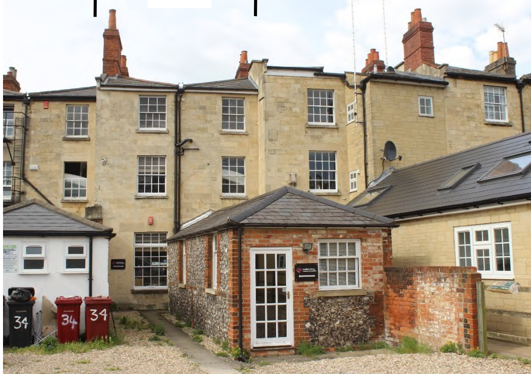
Figure 2 Rear elevation of No. 36 with the single storey outbuilding.
