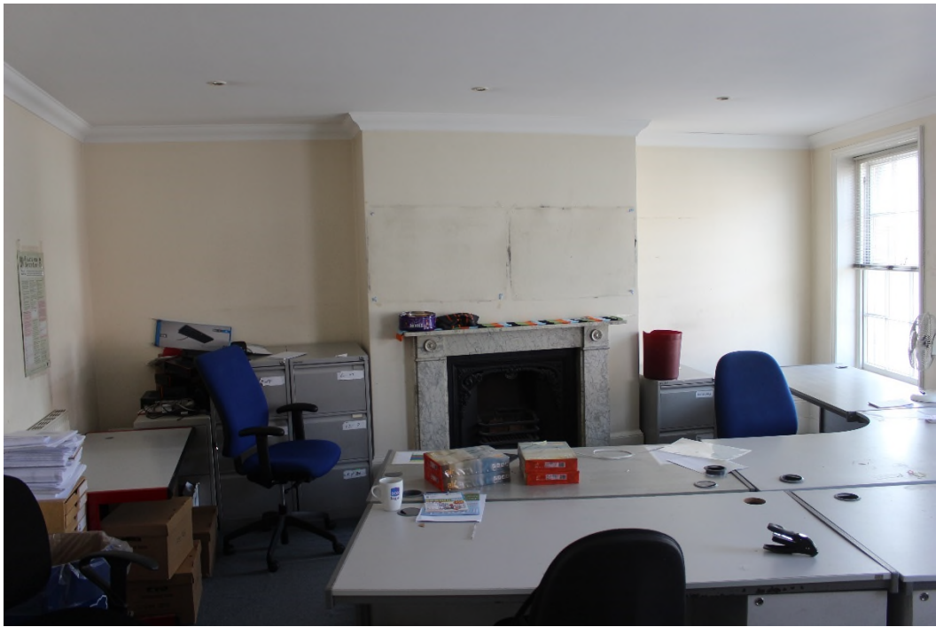
Figure 8 Front first floor room.
