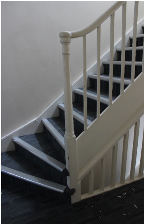
Figure 6 Stairs from ground to first floor – lower part showing the newel post.
