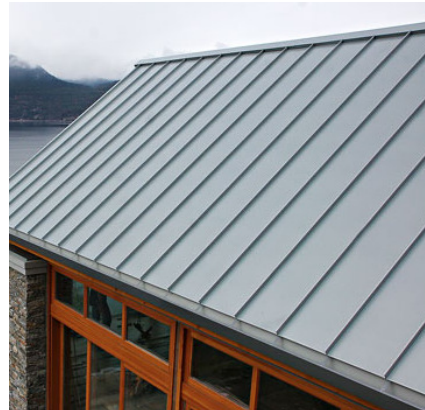
Example of standing seam zinc roof
