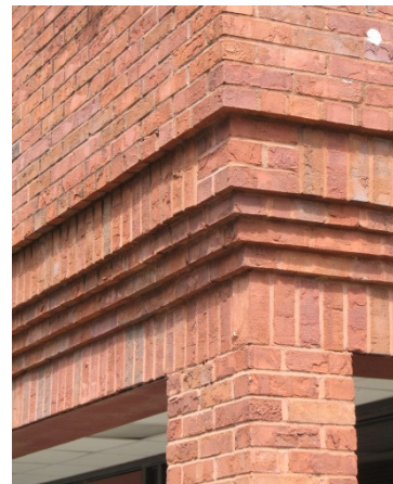
Stepped brickwork as proposed for corner tower
