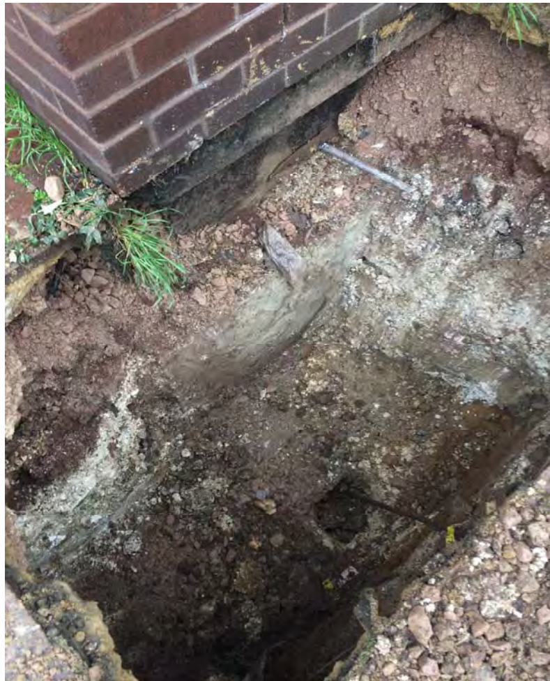
View of foundations and services encountered in Trial Pit No 2
