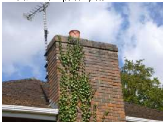
9. Lead flashing at base of chimney tight to tiles.
