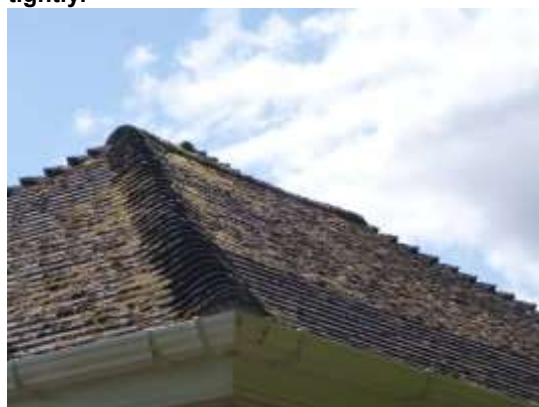
6. Tightly fitted moss covered tiles on garage.
