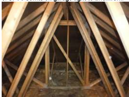
10. Floor of roof void covered with fibreglass.
