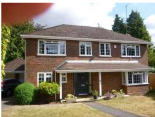
1. Front of house viewed from south-west.
