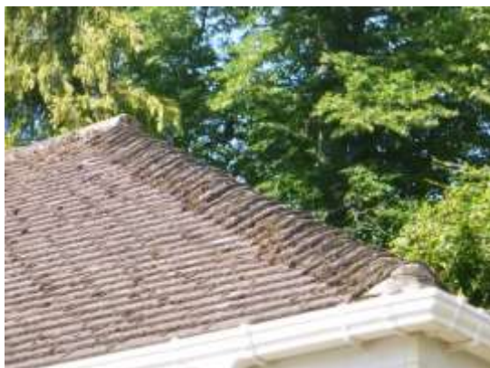
7. Mortar under hips complete.
