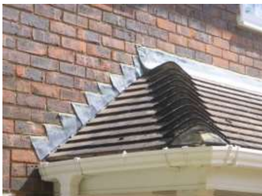
3. Lead flashing fitted tightly around canopy.
