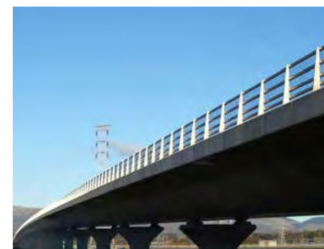
(Images: Stel Construction Info.)
