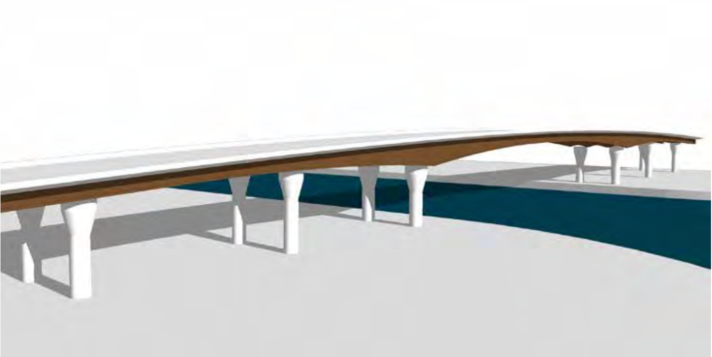
Tapering depth steel girder with open abutments. The bending moment permits a shallower girder at the apex of the bridge.
