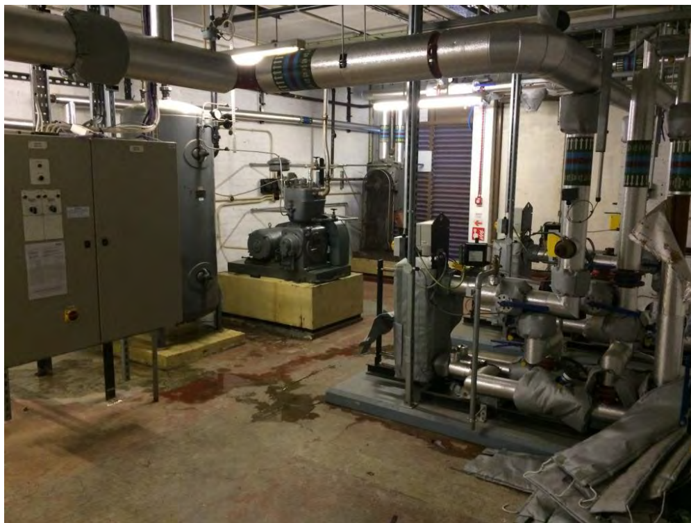
Photo 4 – Plant room in basement. All machinery on raised plinths. Some water on floor, no visual or olfactory evidence of contamination.
