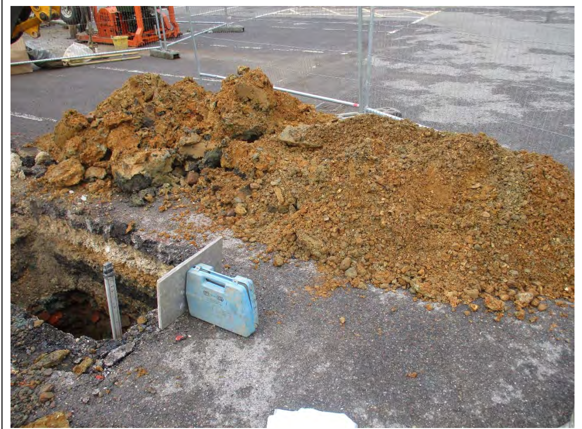
Trial pit: TP02 spoil
