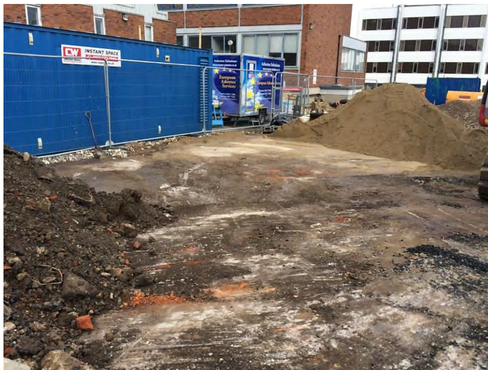
Photo 7 – Site of BH03 in former car park. Currently a contractor compound. Despite scraping away spoil piles the well could not be located.
