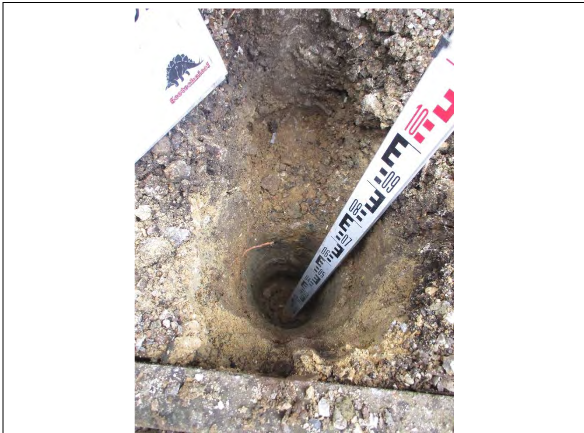
Inspection pit: IP01
