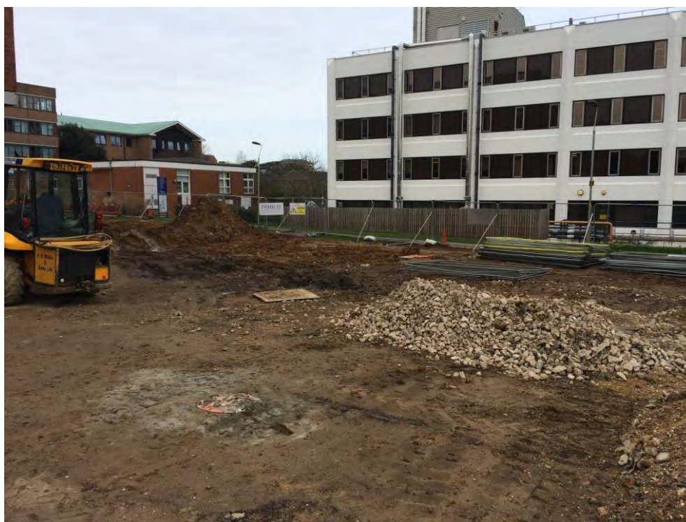
Photo 6 – Site of BH02 to the north of the Engineering building. Contractor confirmed excavation of this well during subsurface utility re-routing/installations.
