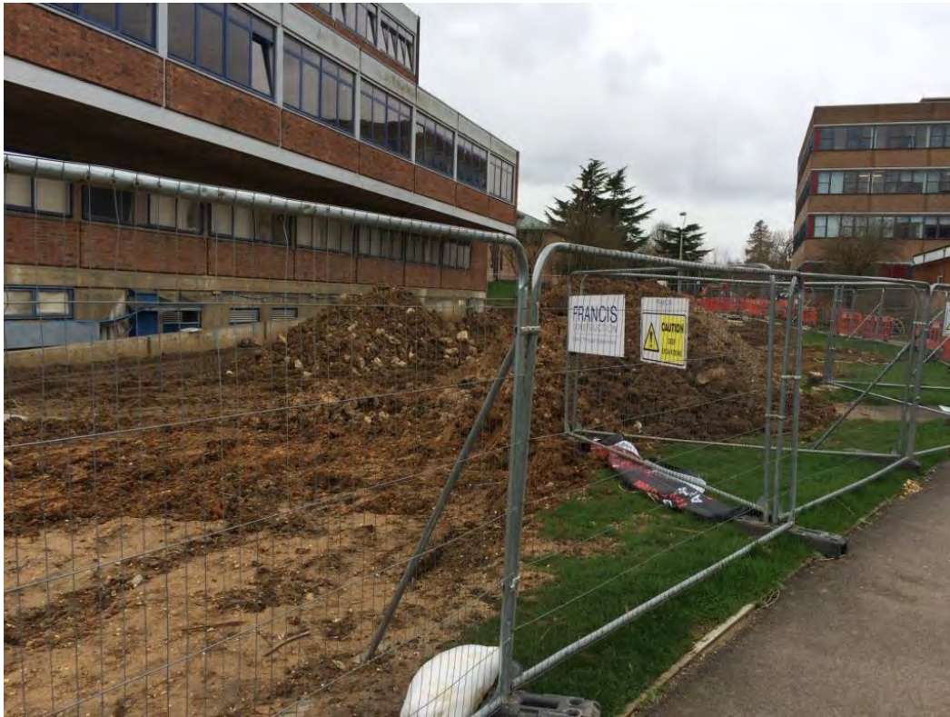
Photo 11 – View south-west to Engineering building from pathway to north.
