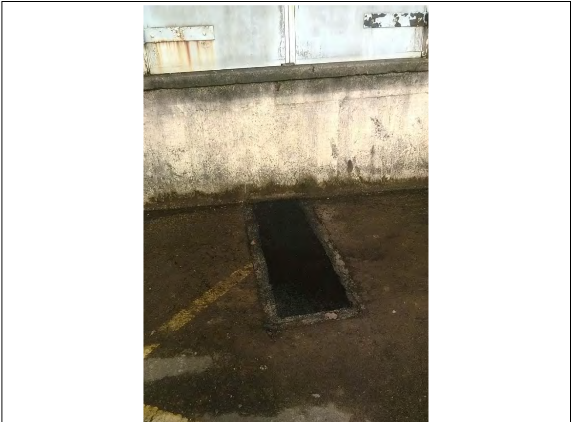
Inspection pit: IP02 reinstatement
