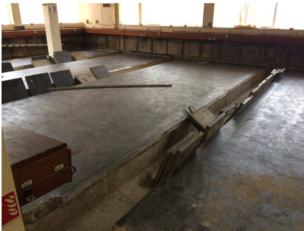
Photo 2 – Service ducts on ground floor of single storey south section. Asbestos removed from ducts, no visual olfactory evidence of contamination.
