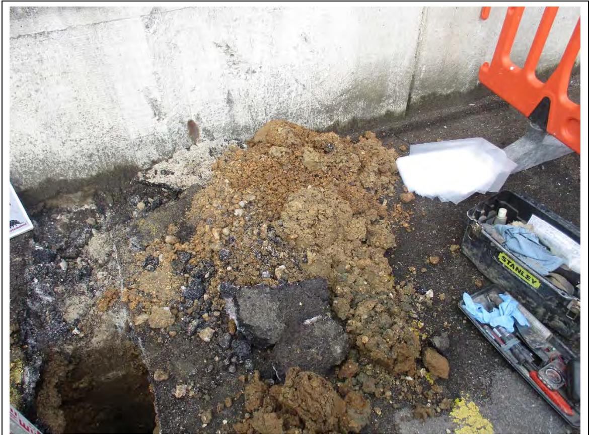
Inspection pit: IP02 spoil
