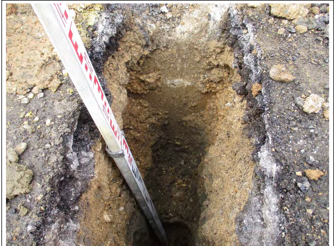
Inspection pit: IP02 profile
