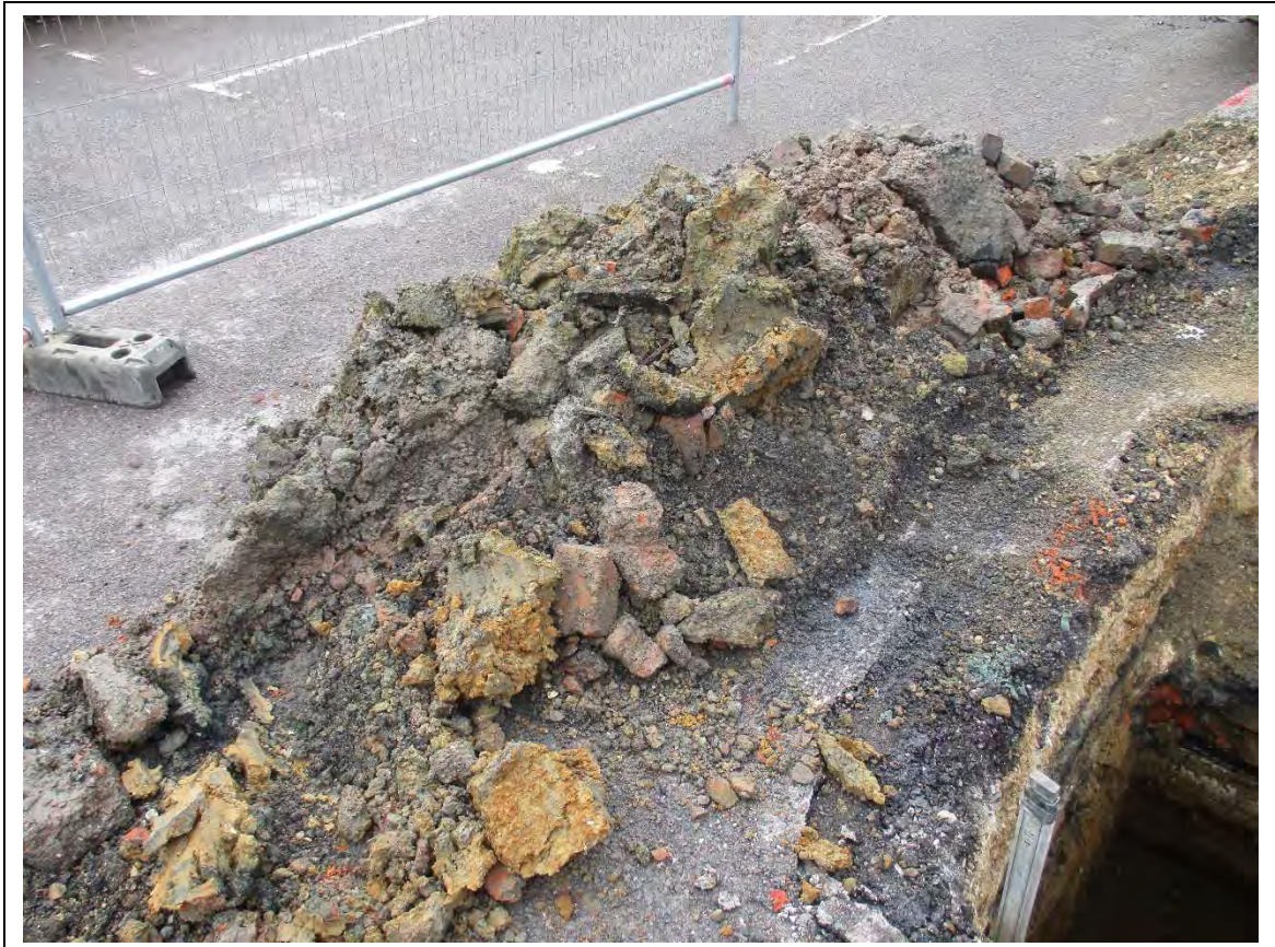
Trial pit: TP02 spoil
