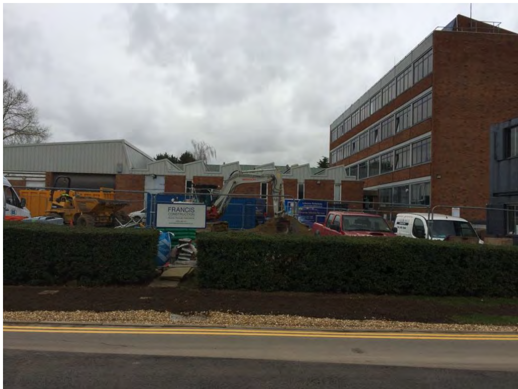
Photo 10 – View west to Engineering building from campus road to east.
