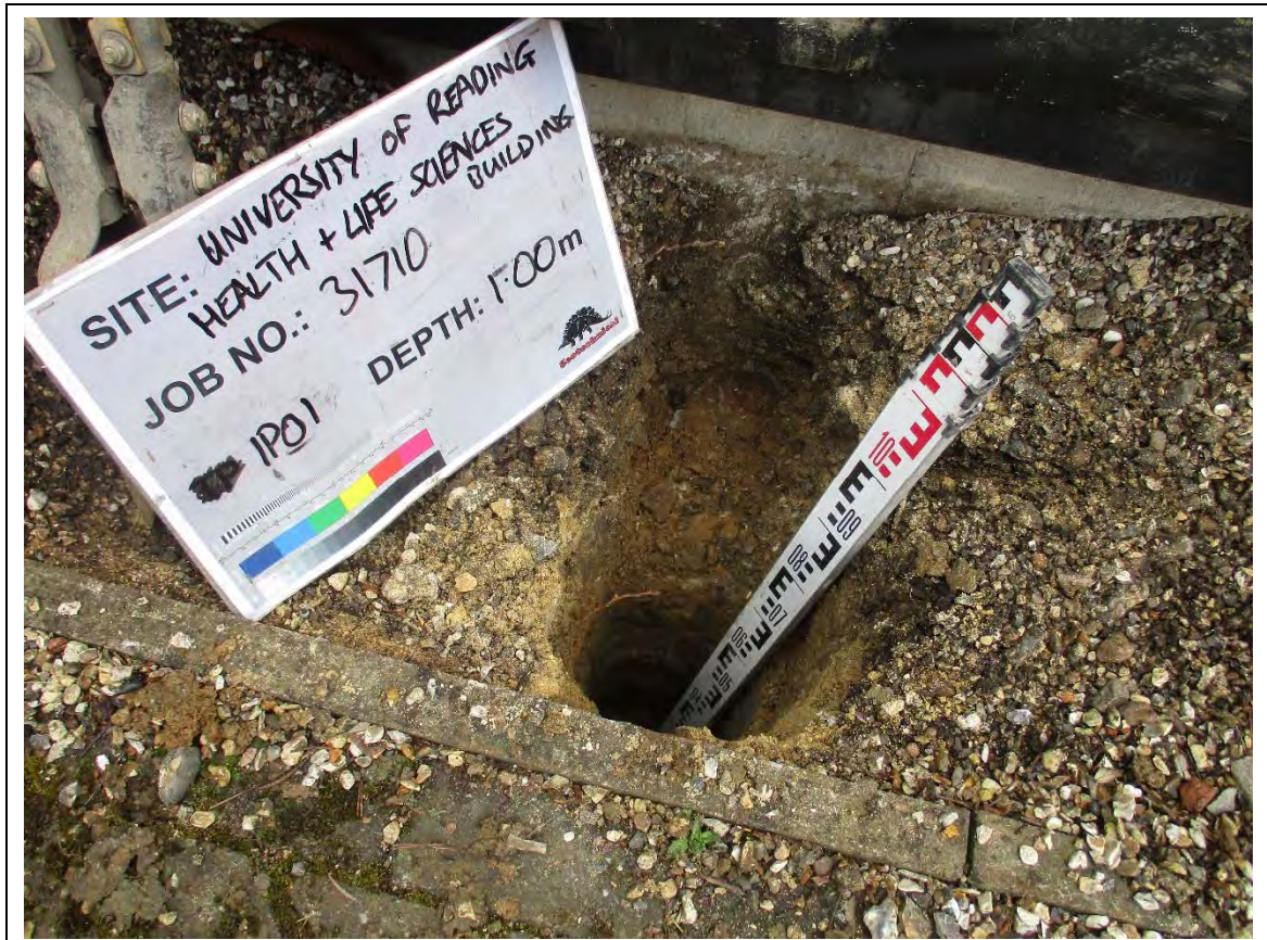
Inspection pit: IP01
