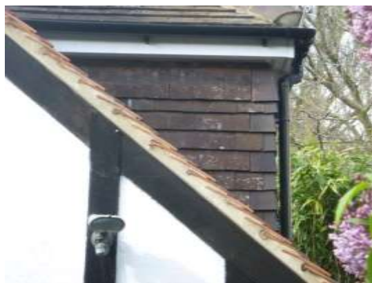
10. Verge tiles mortared fully on the front gable end.
