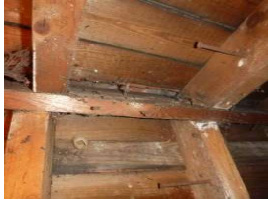
14. Roof tiles exposed at the ridge.
