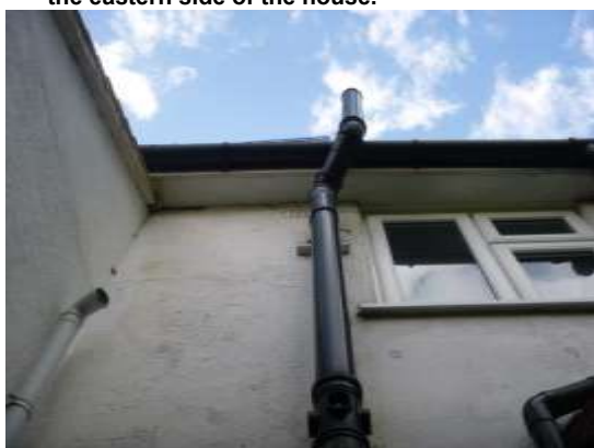
11. Soffit boxes tight around the eaves of the house.
