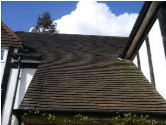
3. Roof tiles mostly tightly fitted to the front of the house; slight gaps beneath verge tiles.
