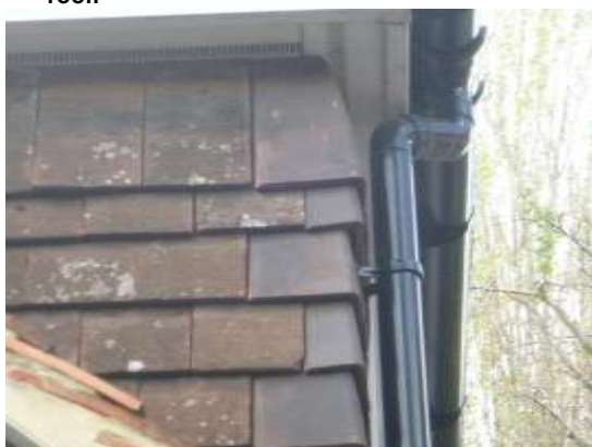
9. Corner hanging tiles lifted on the hipped roof to the eastern side of the house.
