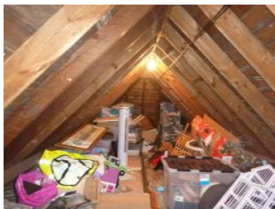
12. Internal view of the roof space viewing west.
