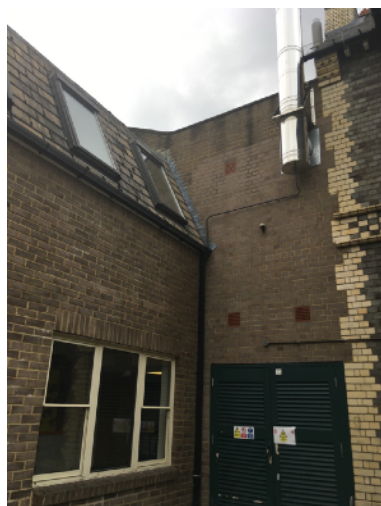
Figure 6. Rear of building (S)
