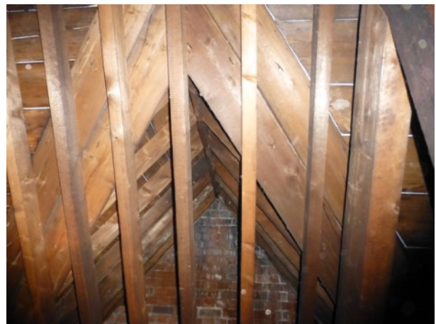
Figure 7. West roof void with struts
