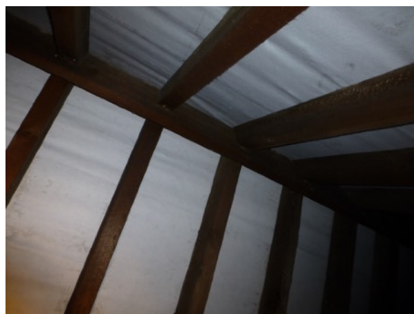
Figure 9. Ridge of area of E roof void
