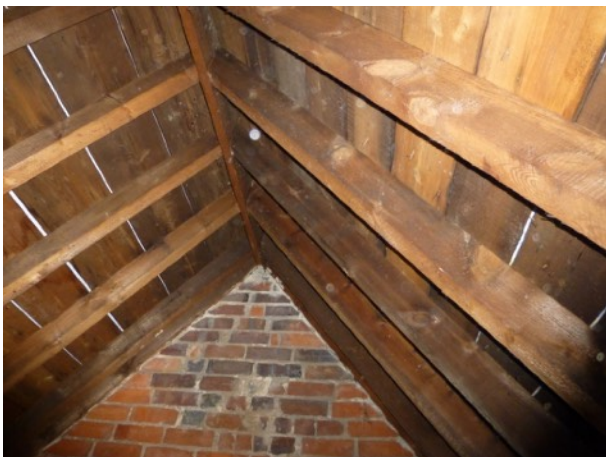
Figure 6. West roof void of building
