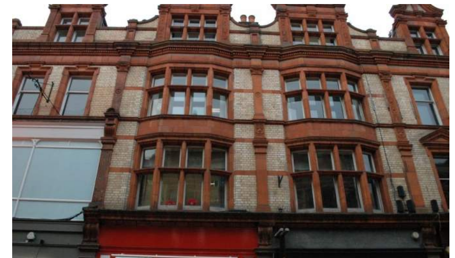
Plate 15: Front façade of 17 Queen Victoria Street
