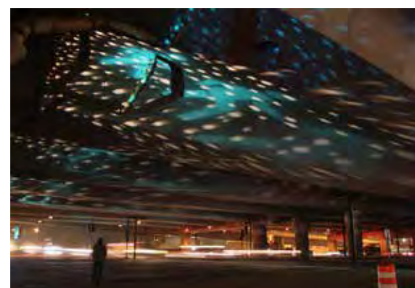
Figure 102. I-93 Lighting Project, Boston Mas.
