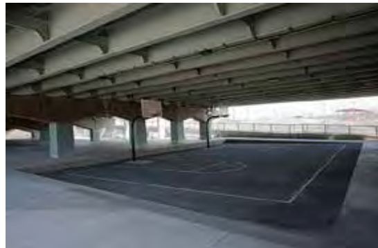
Figure 94. Games courts, Underpass park, Toronto
