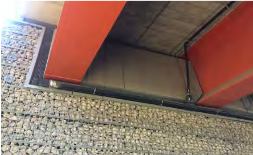
Figure 118. Example of weathering steel beam meeting abutment
