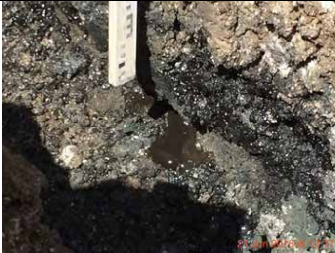
Photograph 13 – Free phase product identified to be emanating from the end of a deep surface water drain within STP11. The surrounding material was also grossly contaminated.
