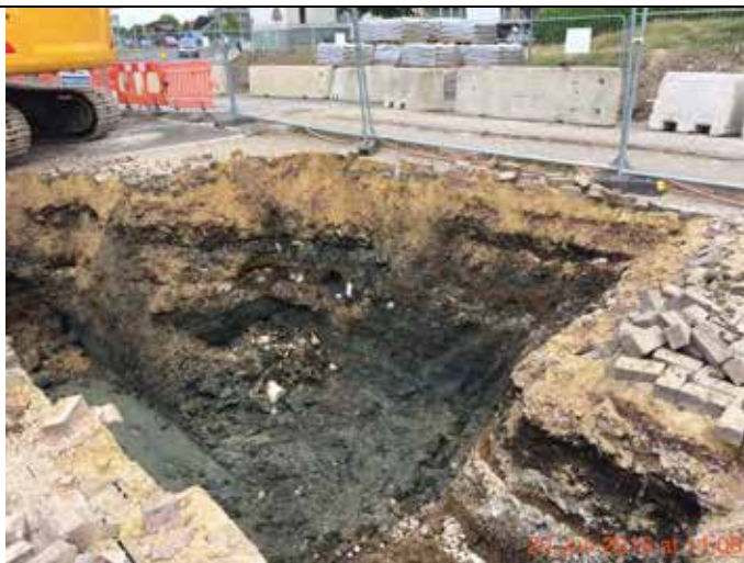
Photograph 9 – Completed extent of STP5 once all timbers had been removed.
