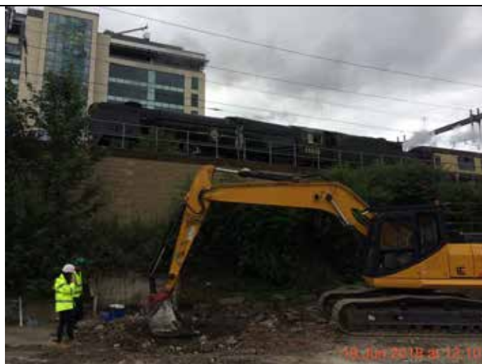
Photograph 3 – Advancement of STP1 in the south of the site.
