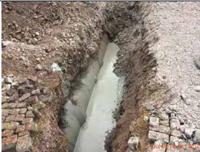
Photograph 40 – Grout pumped from mixing unit into the excavated trench until filled to approximately halfway up the culvert edge.
