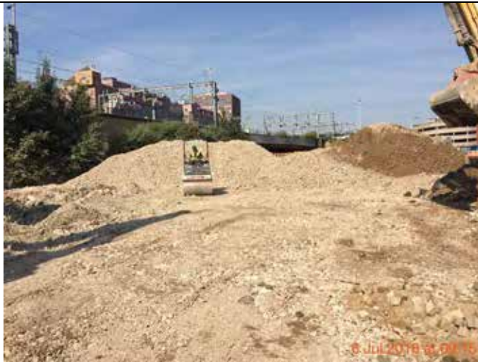
Photograph 34 – Eastern half of the remedial excavation backfilled and compacted with the roller.
