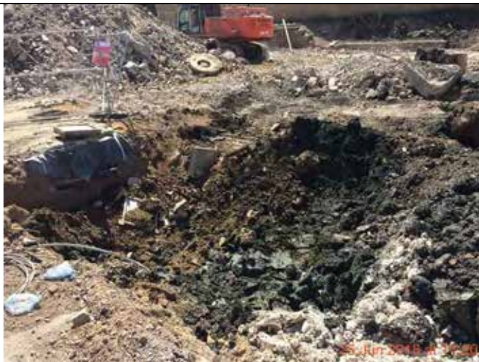
Photograph 17 – View of the area after the removal of the interceptor.
