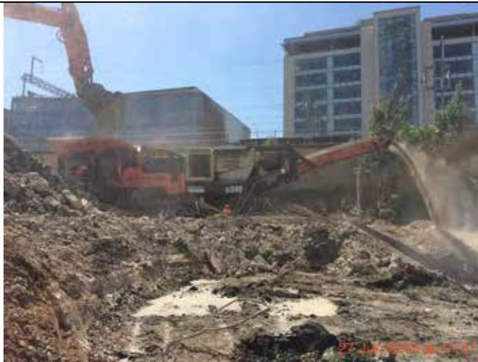
Photograph 22 – Demolition contractor's crusher backfilling directly into the completed remedial excavation.
