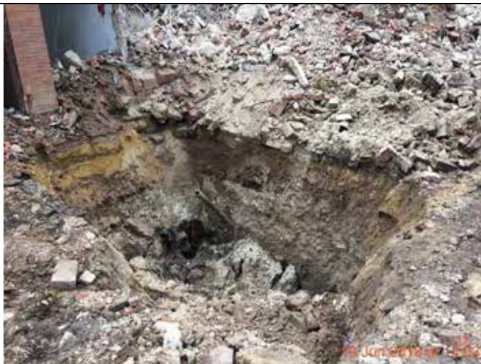
Photograph 5 – Advancement of STP3 in the east of the site.
