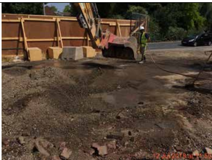
Photograph 48 – Soilfix plant / personnel locating BH2 for the groundwater sampling round.
