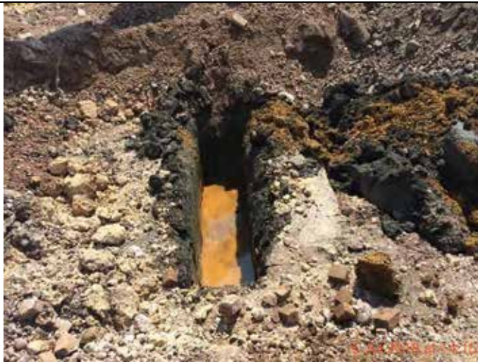
Photograph 31 – Deeper trench excavated into the sands and gravels. No free phase product identified.
