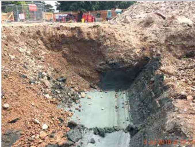
Photograph 29 – View of the eastern excavation area.
