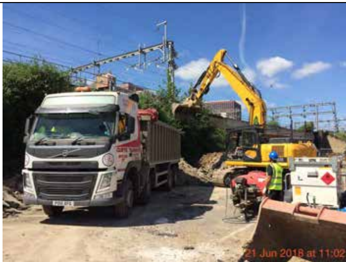
Photograph 14 – 360° excavator used to load stockpiled material into 8-wheel tipper lorries for off-site disposal.
