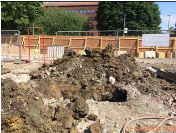
Photograph 47 – Trial pits excavated along the eastern side of the culvert.
