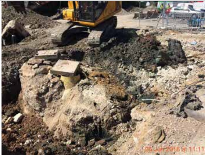
Photograph 16 – View of the southern interceptor prior to removal with surrounding material excavated.
