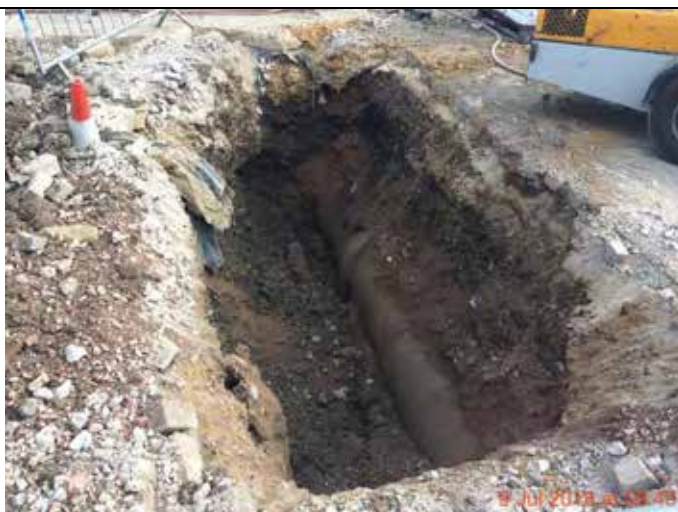
Photograph 36 – Edge of the western culvert exposed prior to construction of the slurry wall.
