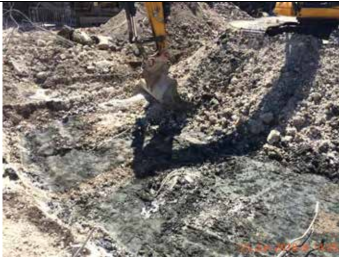
Photograph 19 – Excavation advanced southwards towards the location of STP11.
