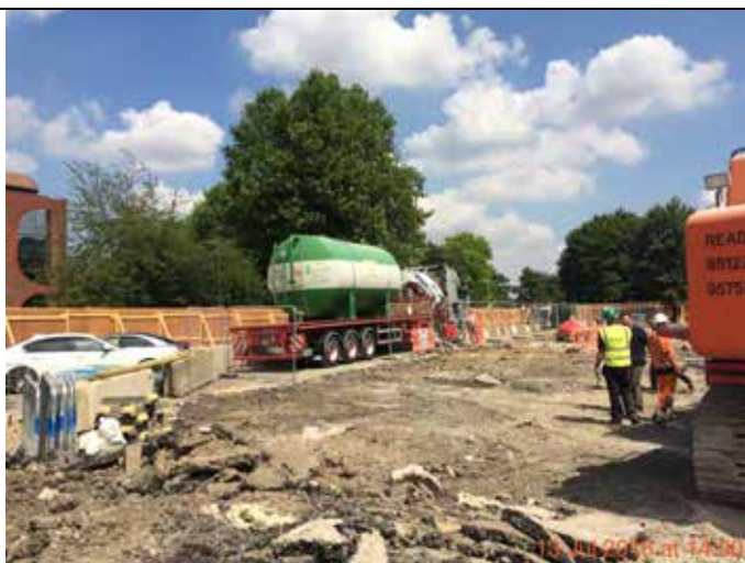
Photograph 54 – Header tank demobilised from site.
