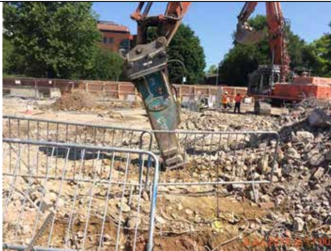
Photograph 25 – Slab and below ground obstructions removed by the demolition contractor.
