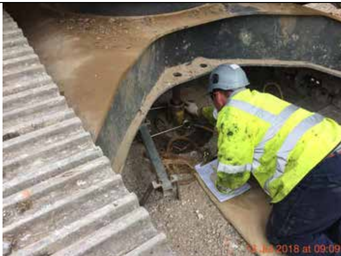
Photograph 50 – Plate bearing tests undertaken.
