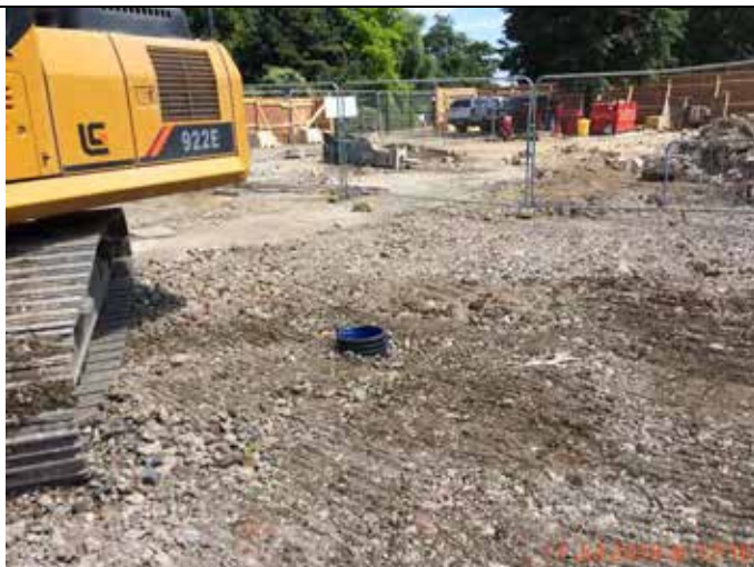
Photograph 45 – Sump New 1c installed.
