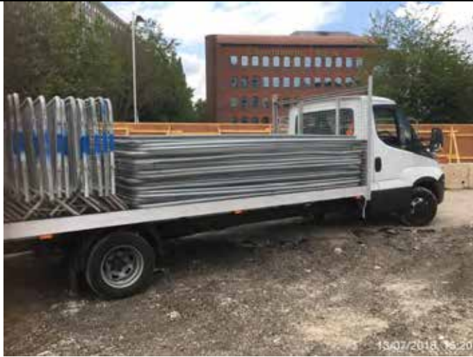
Photograph 55 – Fencing demobilised from site.
