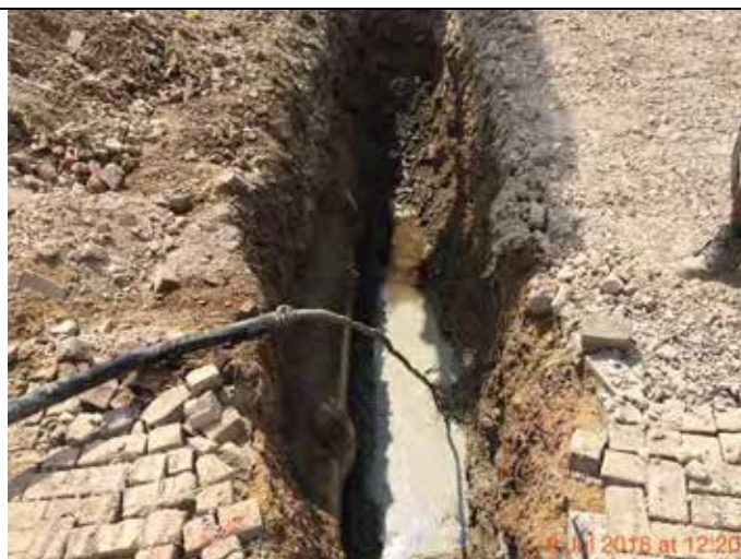
Photograph 39 – Grout pumped from mixing unit into the excavated trench.
