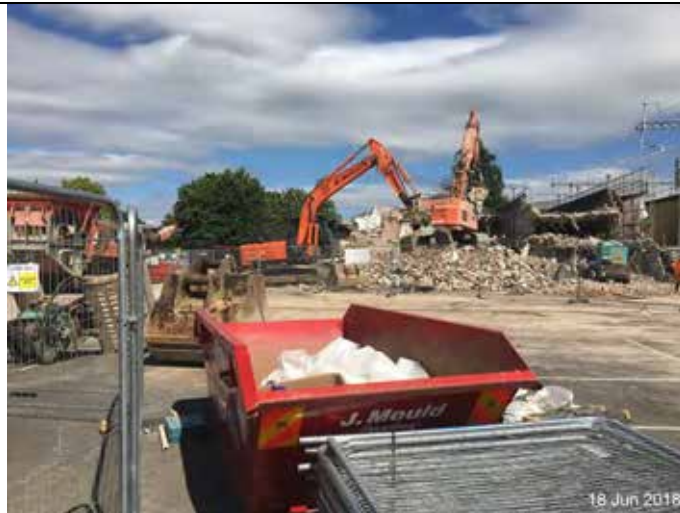
Photograph 1 – View of the delineation / remediation areas upon Soilfix mobilisation to site.
