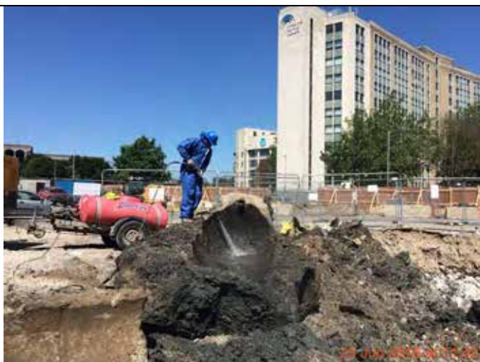
Photograph 18 – The concrete previously encasing the interceptor and removed piles were pressure washed to remove residual free phase product.
