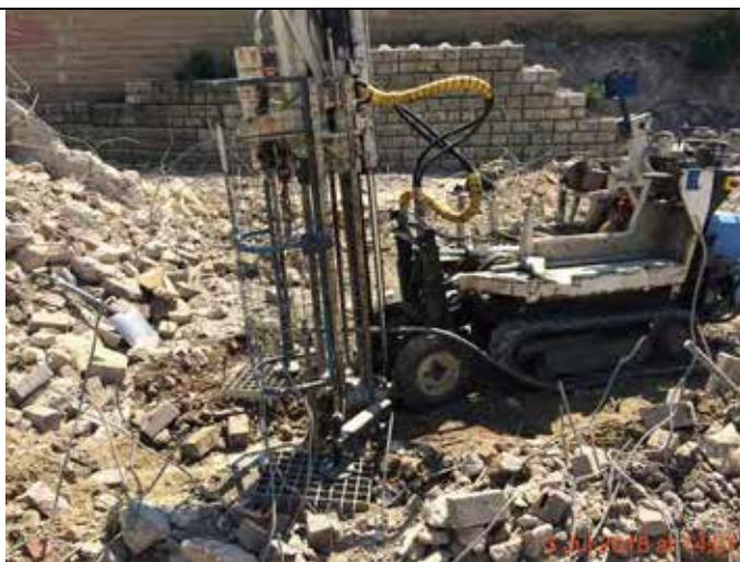
Photograph 27 – Specialist contractor (Tor Drilling Ltd) mobilised to site to undertake grout injection works.
