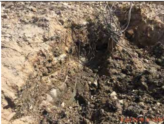
Photograph 35 – Edge of the western culvert exposed prior to construction of the slurry wall. Below ground obstructions requiring removal at this point.
