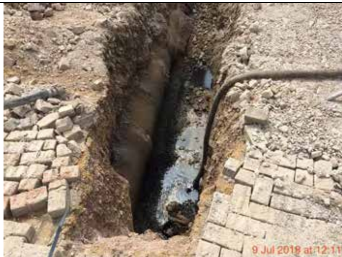
Photograph 38 – Free phase product mobilised from the culvert bedding material at points was removed by a pump to the on-site header tank.
