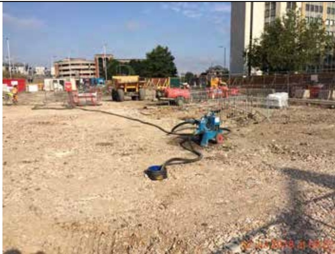
Photograph 46 – Groundwater pumped from sumps into the on-site header tank.
