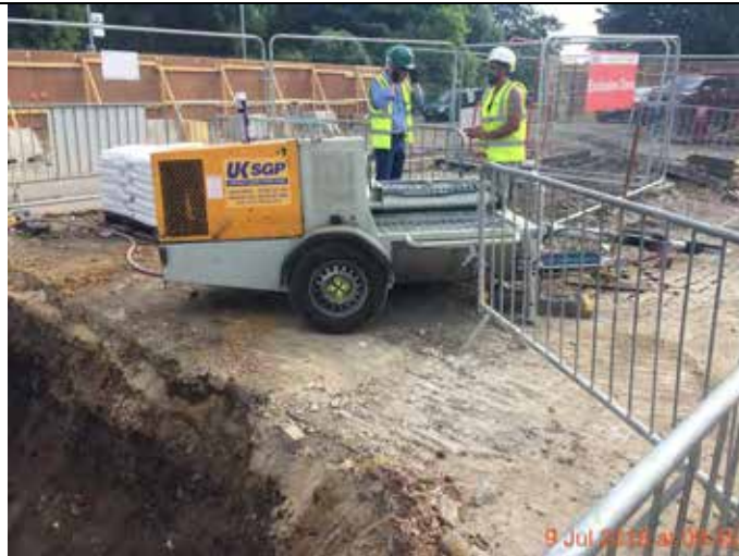
Photograph 37 – Slurry batching equipment mobilised to site.
