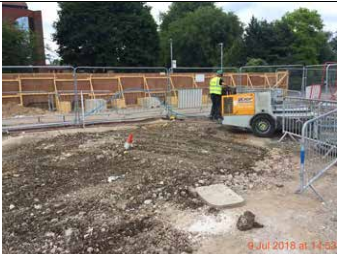
Photograph 41 – Slurry wall left to cure for a period and backfilled with arisings.
