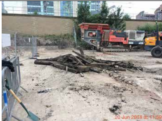
Photograph 10 – Creosote impacted timbers that were removed.
