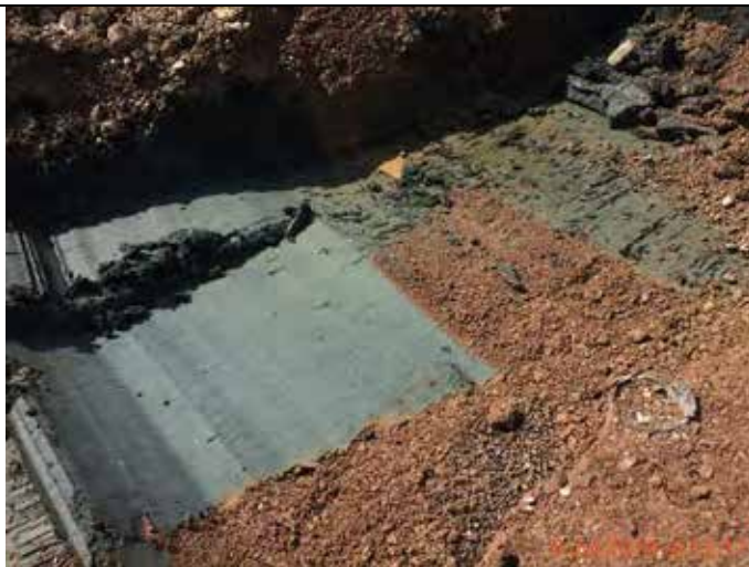
Photograph 32 – Deeper section of impacted alluvium excavated in the northeast corner of the excavation.
