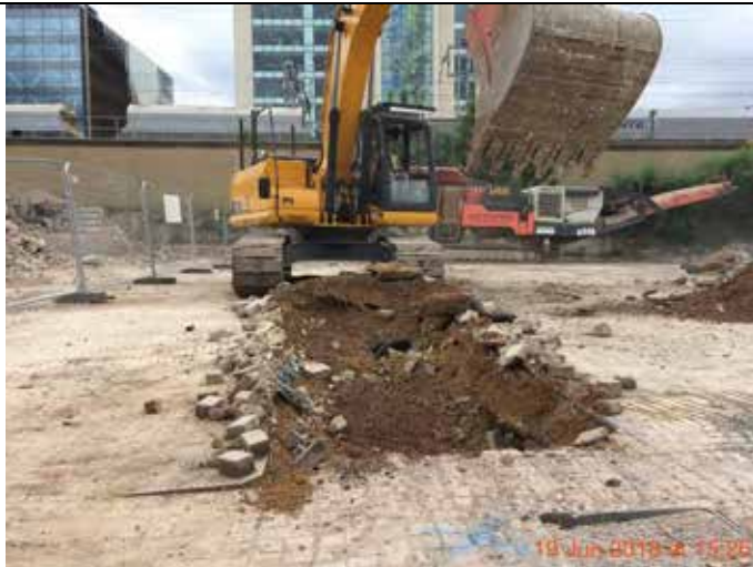
Photograph 7 – Advancement of STP4.
