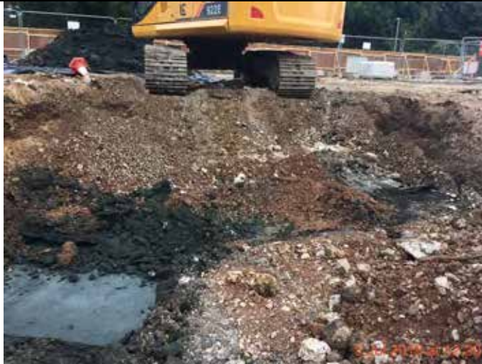
Photograph 28 – View of the eastern excavation area.
