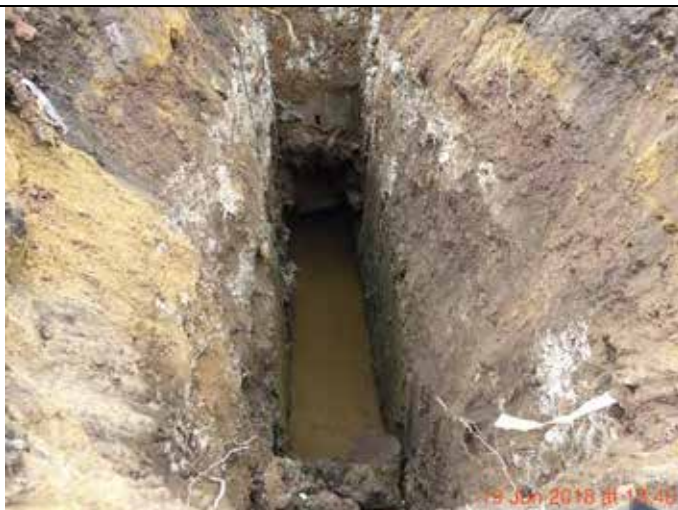
Photograph 6 – View of the groundwater surface within STP3. No free phase product visible.
