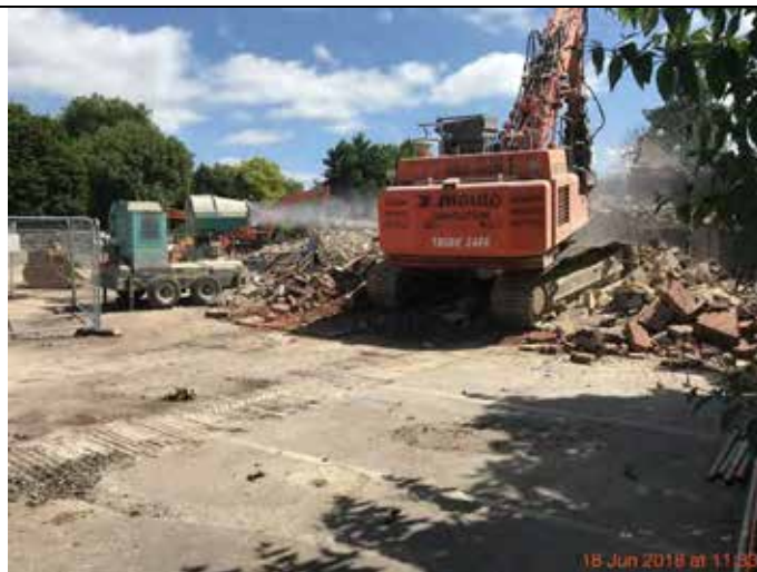
Photograph 2 – View of the delineation / remediation areas upon Soilfix mobilisation to site.
