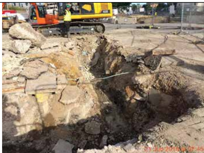
Photograph 12 – Advancement of STP6.
