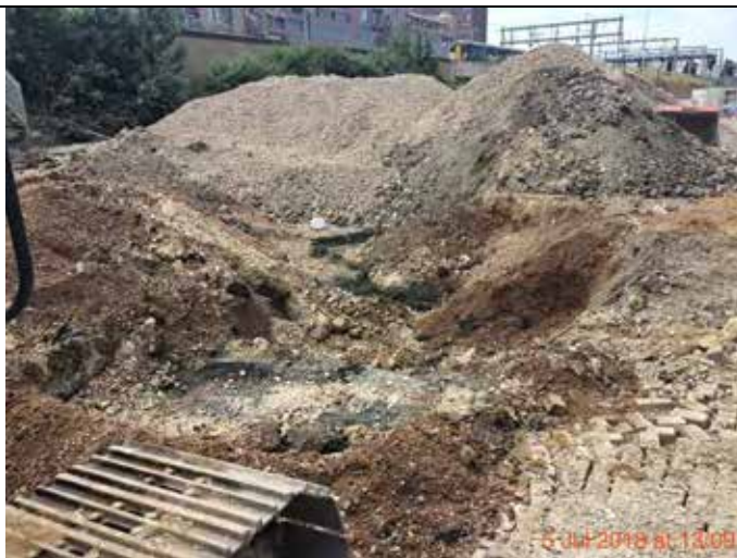
Photograph 30 – View of the eastern excavation area.
