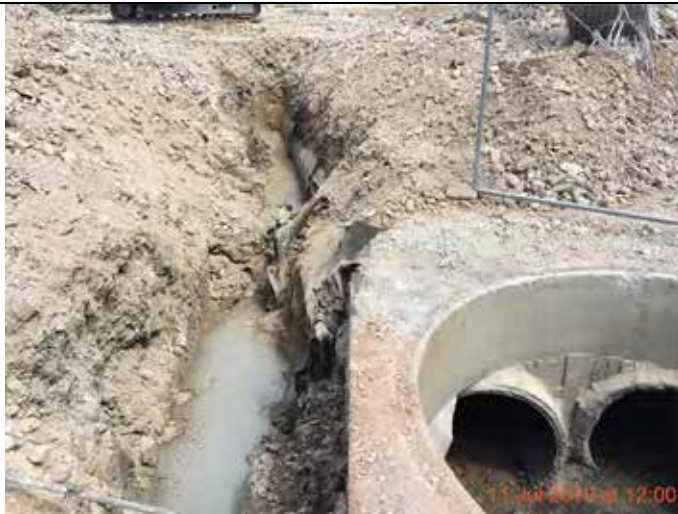
Photograph 43 – Trench excavated up to this location, where the contaminated culvert bedding material terminated. The slurry wall constructed up to this point.
