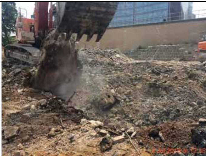
Photograph 26 – Below ground obstructions removed by the demolition contractor.
