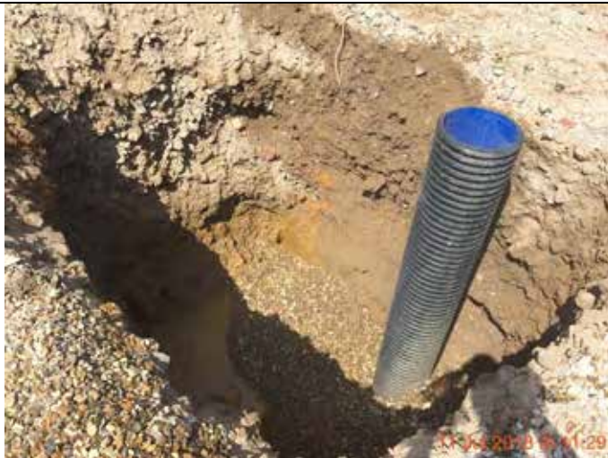
Photograph 44 – Sump New 1c installed for the upcoming groundwater sampling rounds.
