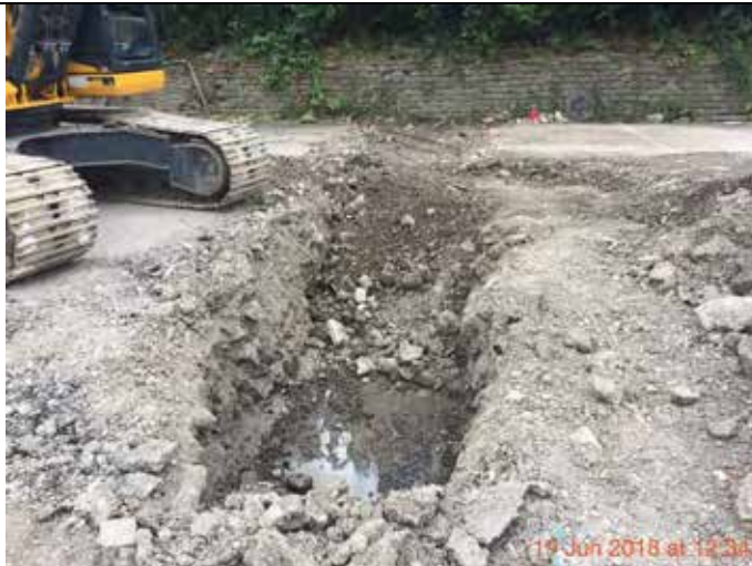
Photograph 4 – Advancement of STP2 in the south of the site.
