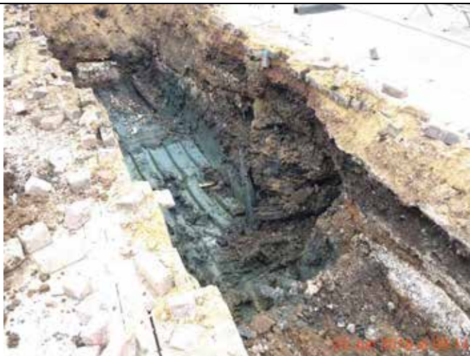
Photograph 8 – Advancement of STP5. Creosote impacted timbers discovered from circa 1.1m bgl and running out of the initial excavation face, requiring extension of the excavation to remove.
