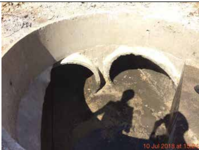
Photograph 42 – Internal view of the construction of the culverts from the southern junction.
