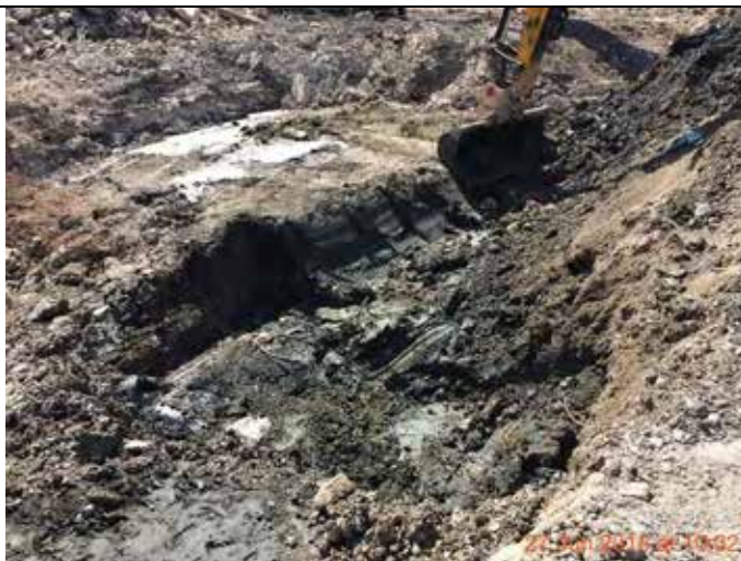
Photograph 21 – View of the western remedial excavation looking southwards. Note the deeper section in the foreground where the deep surface water drainage pipe was chased out.
