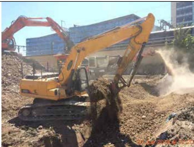
Photograph 23 – Soilfix 360° excavator assisting in moving crushed concrete from the outfall of the crusher belt and spreading over the remedial excavation.
