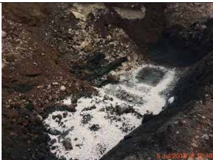
Photograph 33 – ORC pellets applied to the base of the remedial excavation to assist in breaking down any residual hydrocarbon contamination.
