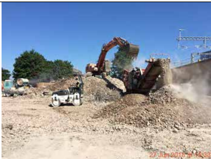
Photograph 24 – Backfilled remedial excavation compacted with a roller.
