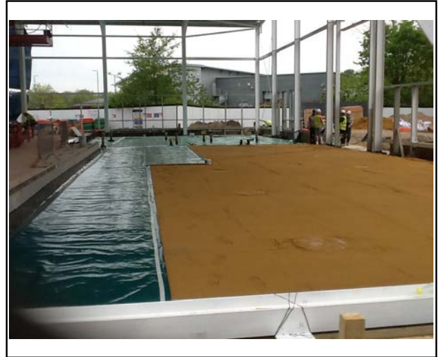
Application on sand blinding
