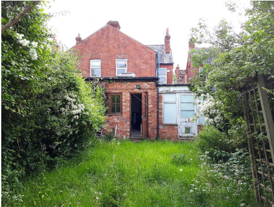
Rear view of 106 Wantage Road
