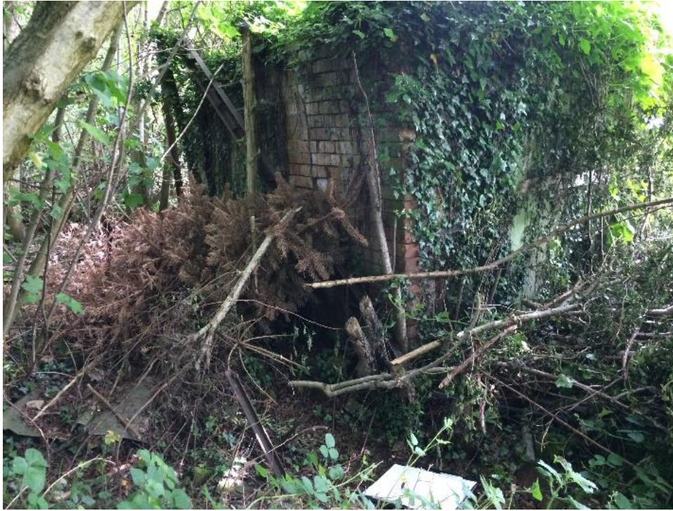
Photo 1: TN1 remains of brick building
