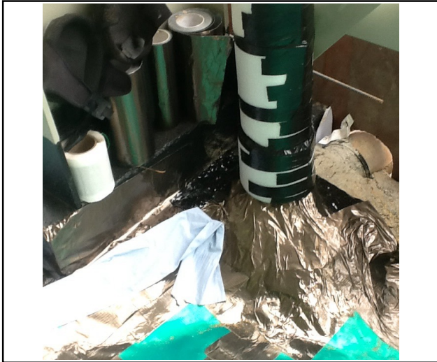
Pipe penetration complete
