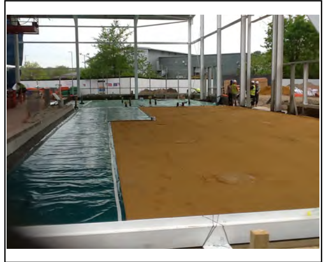
Application on sand blinding
