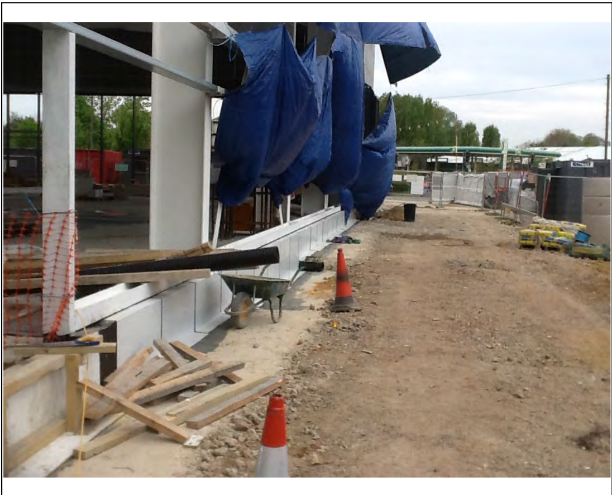
Overview wall A
