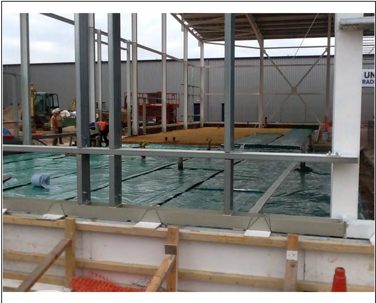
Overview area 7/9 - A-H
