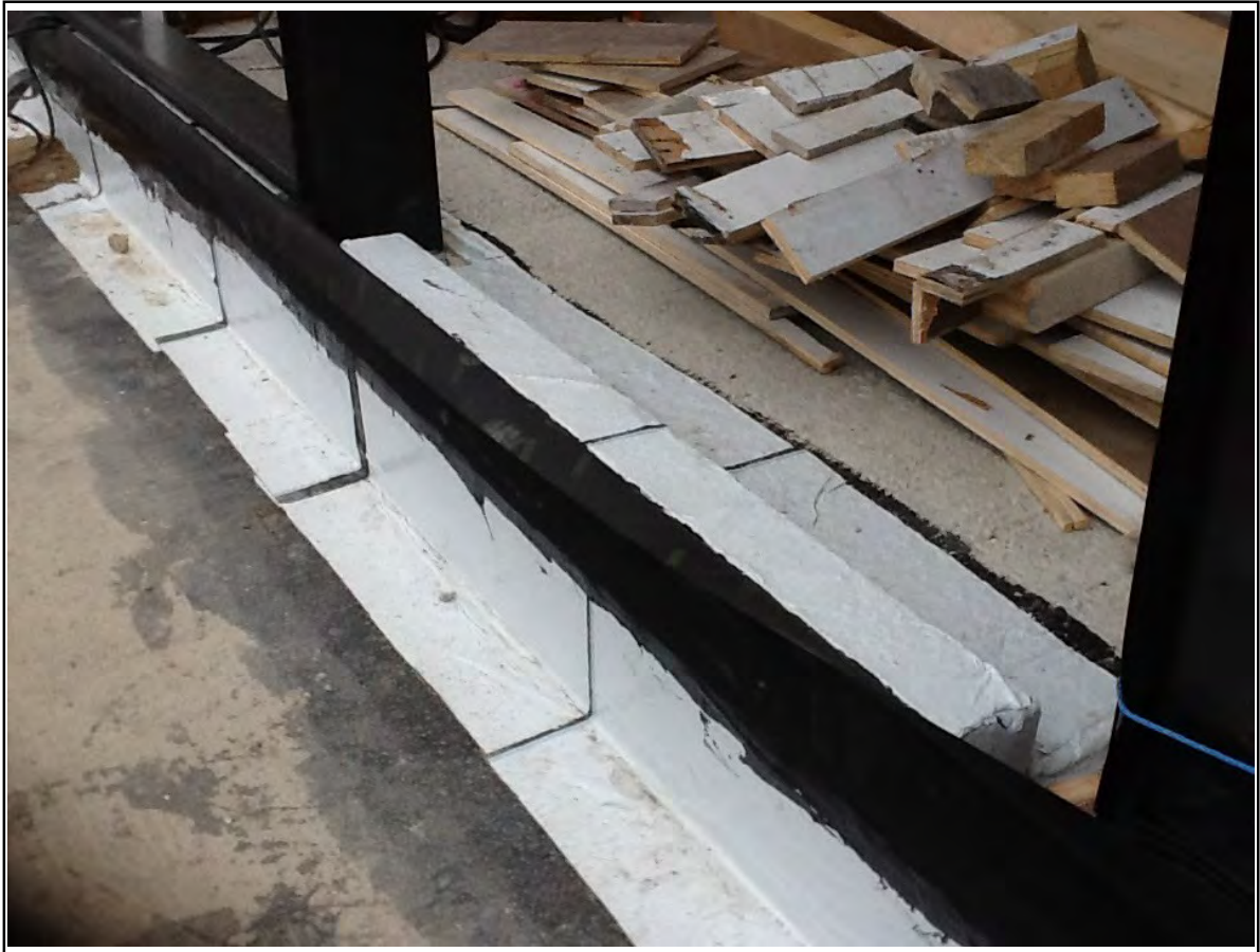
Overview wall A
