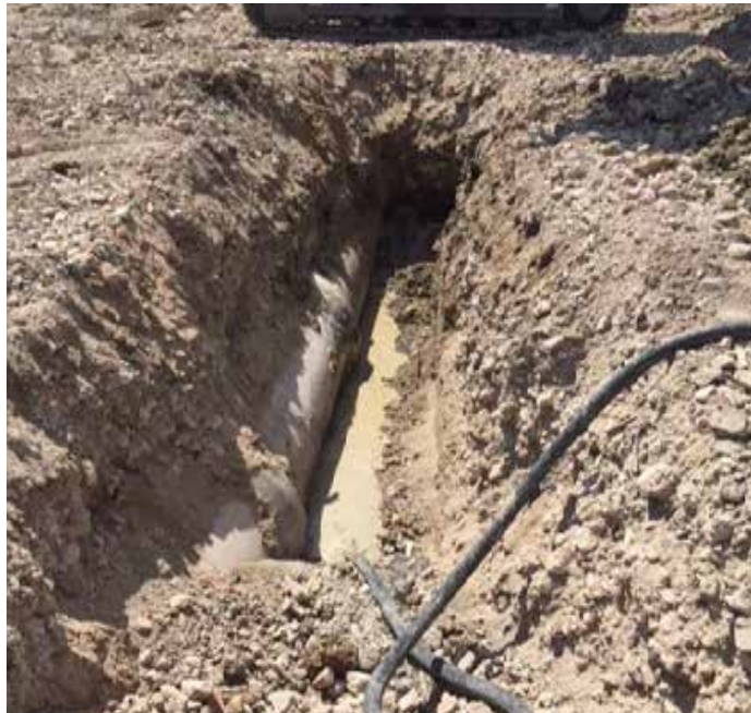
Photo 21. Grouting of culvert in the centre of the site.
