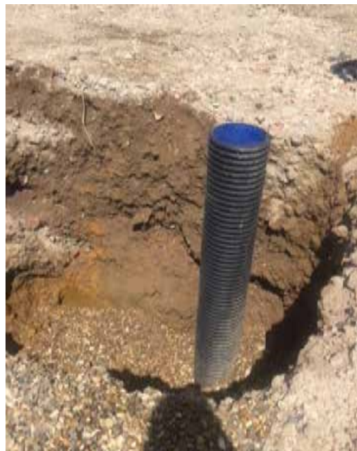
Photo 16. Installation of New Sump 1C
