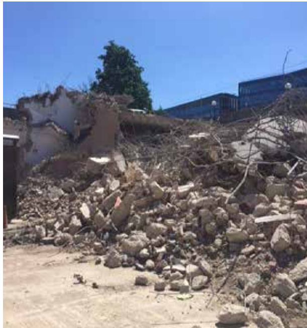
Photo 3. Building during demolition on 19/06/2018
