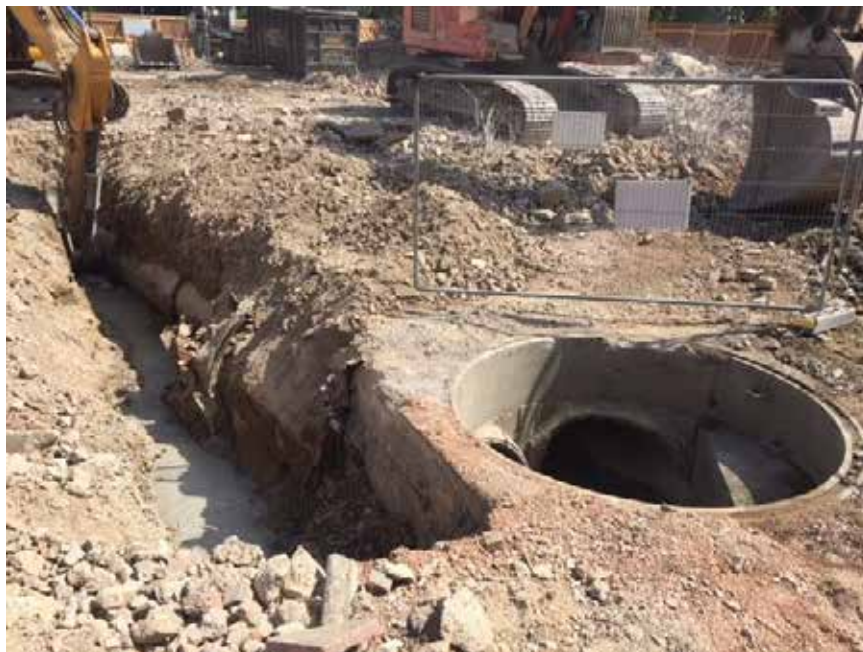
Photo 24. View of grouting works in the south of the site (12/07/2018)
