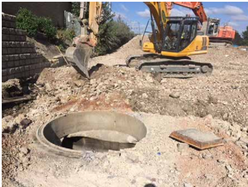
Photo 22. View of the chamber in south of the site
