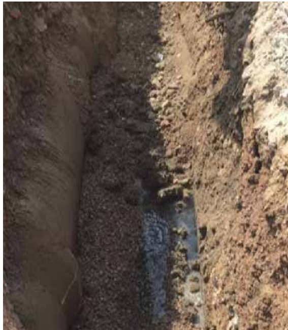
Photo 20. View along east of culvert showing bedding material
