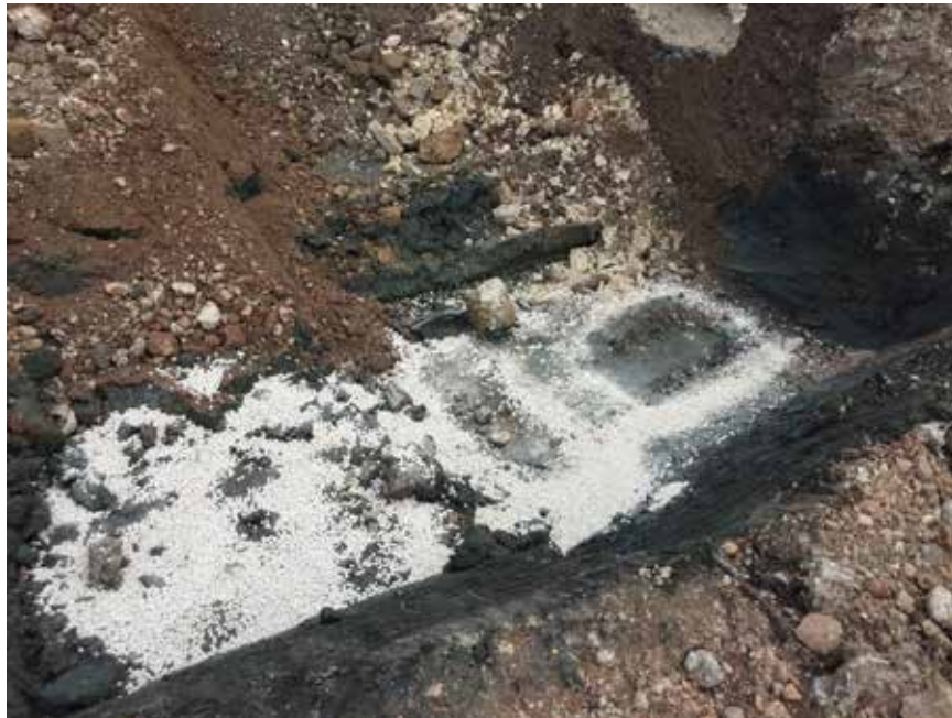
Photo 15. Application of ORC in target areas (05/07/2018)
