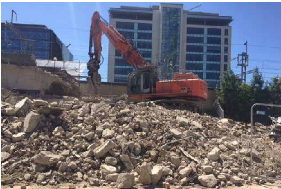
Demolition Material on 18/06/2018
