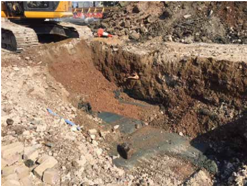
Photo 11. Top of alluvium at validation depth
