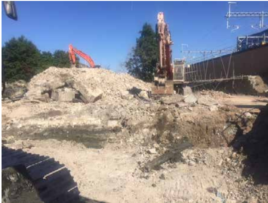
Photo 9. Excavation and stockpile of building material
