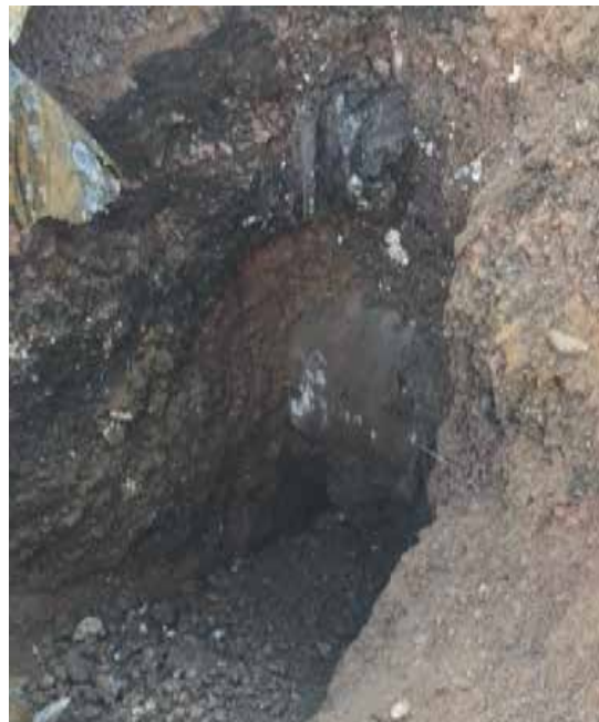
Photo 17. Trial Pit exposing the west of the Culvert
