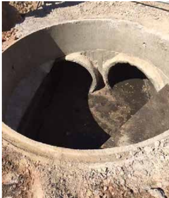
Photo 23. View of both culverts from chamber in the south (10/07/2018)
