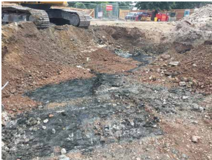
Photo 14. Bulk dig excavation (Area 1)
