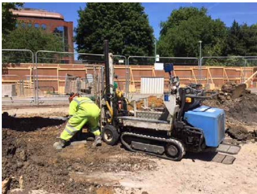
Photo 18. Grout injection works in the north of the site (02/07/2018)
