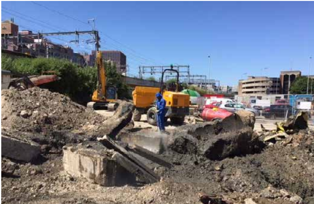
Photo 7. Concrete from around interceptors following removal
