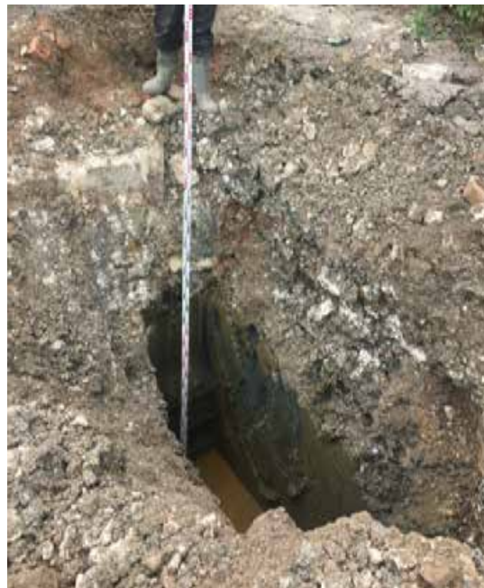
Photo 5. Excavation through alluvium to gravels by BH301 (Edge of STP5)
