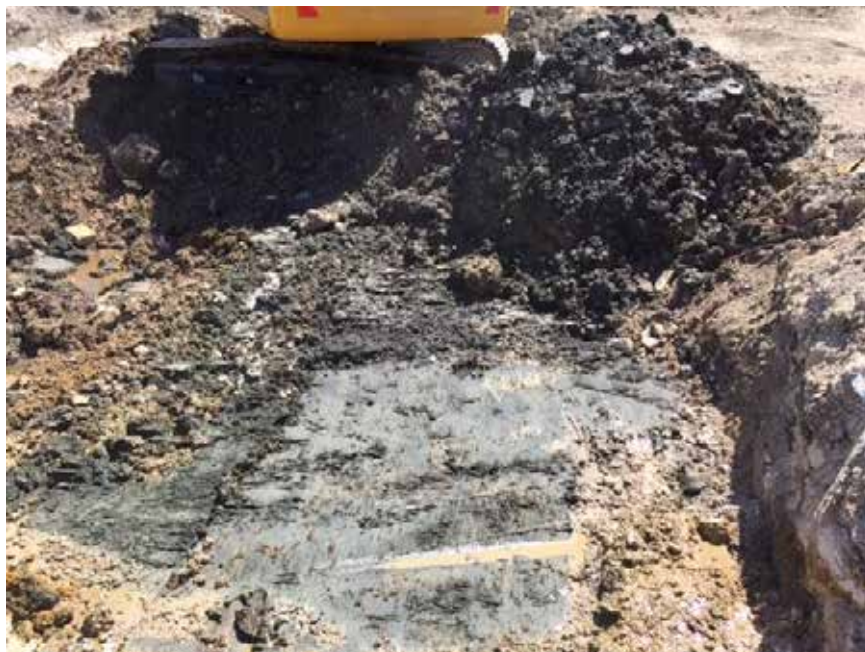
Photo 8. Top of alluvium at validation depth in Area 1
