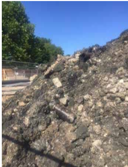
Photo 10. Stockpile of material containing pipe and free product in Area 1
