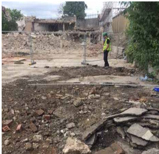
Photo 4. Excavation Location around WS11 on 19/06/2018 (STP 1 & 2)
