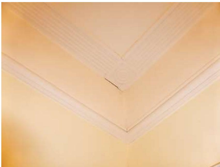
Figure 10: Plaster cornice with reeding and roundel ornamentation
