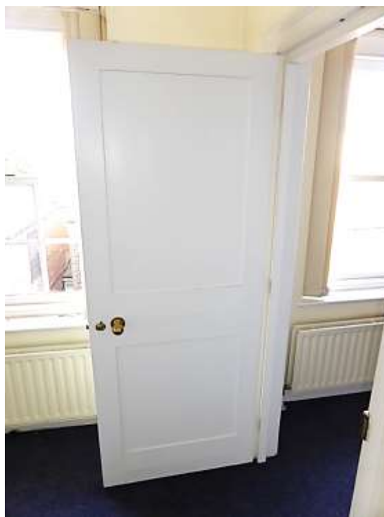
Figure 23: Late 19 th to early 20 th century two panelled door between S4 and S5
