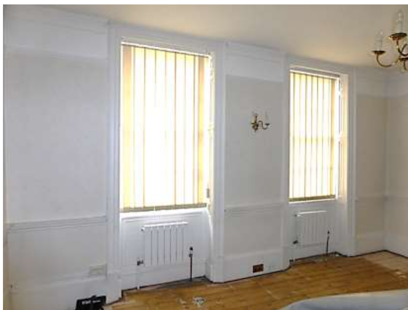
Figure 8: Panelled window recesses with low skirting in G2
