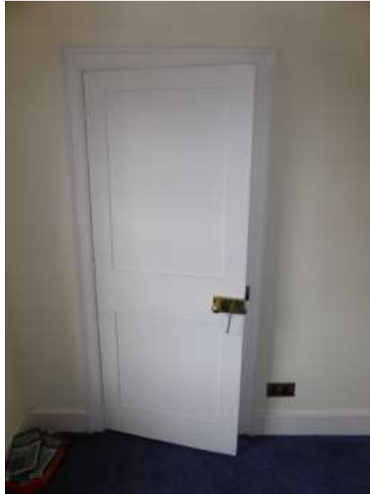
Figure 39: Early 20 th century door in partition between S4 and S5
