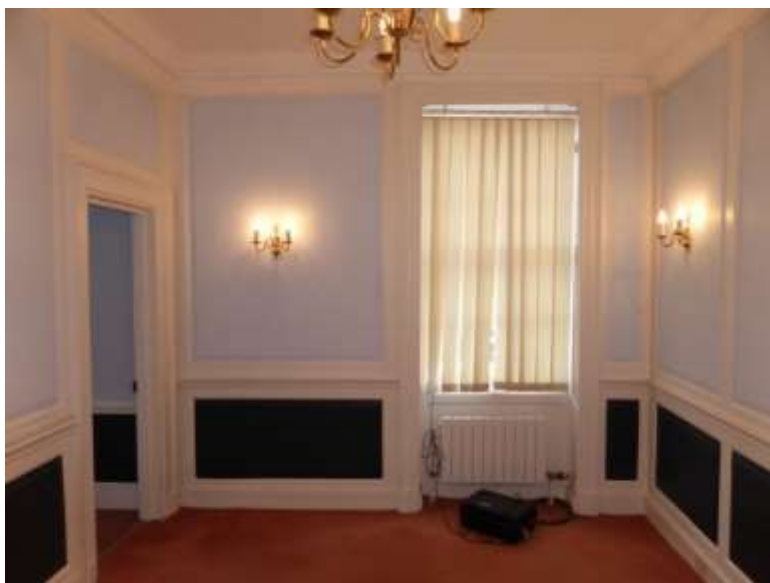
Figure 32: Blocked sash window to the right in F1
