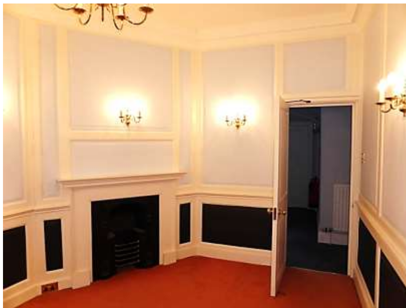
Figure 13: Full-height panelling and corner fireplace in F1
