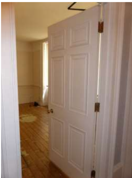
Figure 25: 20 th century six panelled door from the entrance hall (G1) to G2
