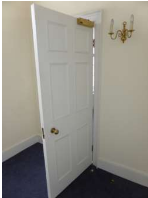
Figure 35: 20 th century six panelled door in the partition between F4 and F5
