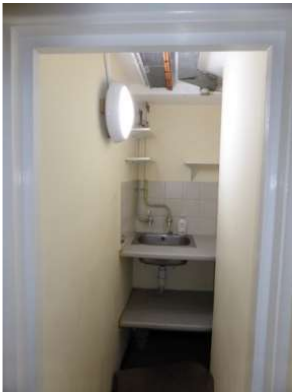
Figure 28: Modern door frame to G4
