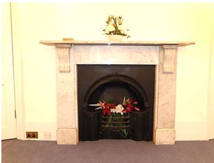
Figure 9: Re-set Victorian fireplace surround and refurbished register grate
