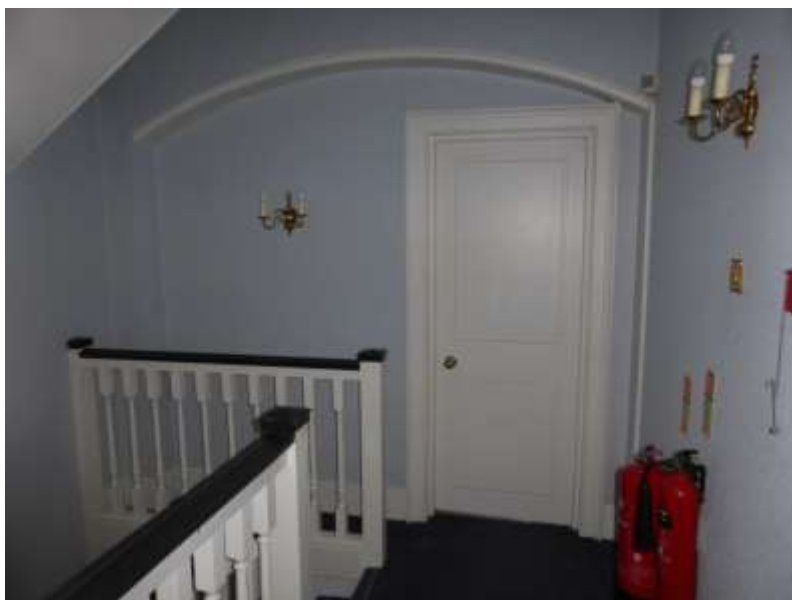
Figure 34: 20 th century door and stud and plaster infill at F4
