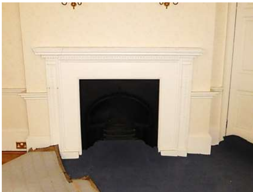
Figure 7: Modified late 18 th century fire surround with refurbished 19 th century register grate in G2
