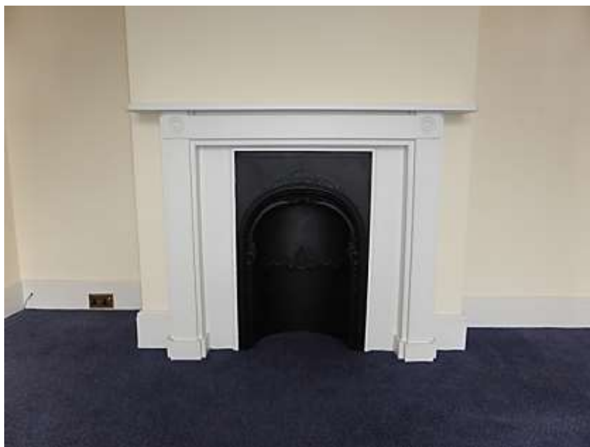
Figure 19: Early 19 th century style fire surround with roundels and refurbished cast iron grate in F5
