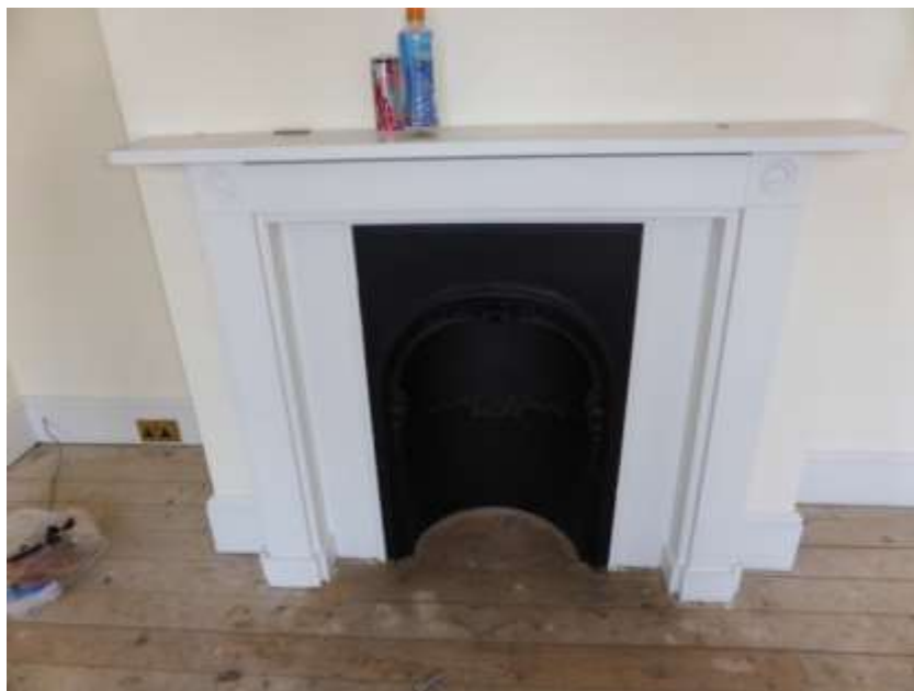
Figure 36: Hearth replaced by floorboards in F5
