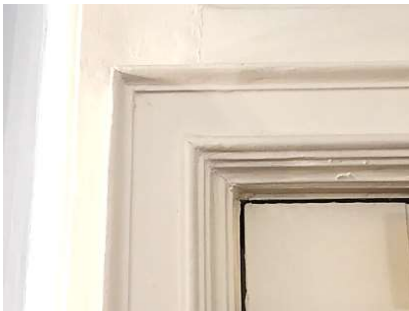
Figure 12: Architrave of door opening between the landing (F3) and F1
