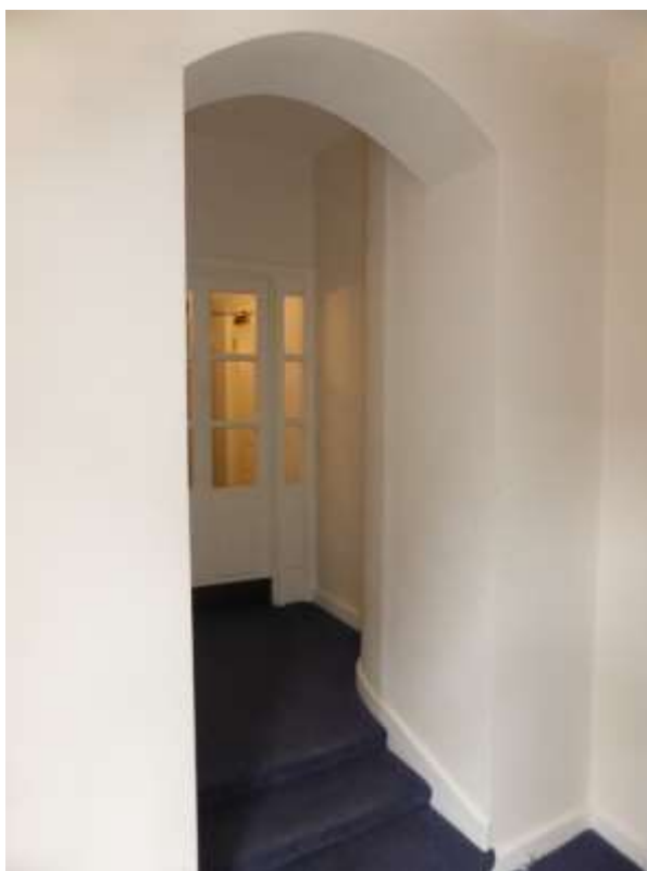
Figure 30: Door opening with segmental arch head at the rear of the entrance hall (G1)
