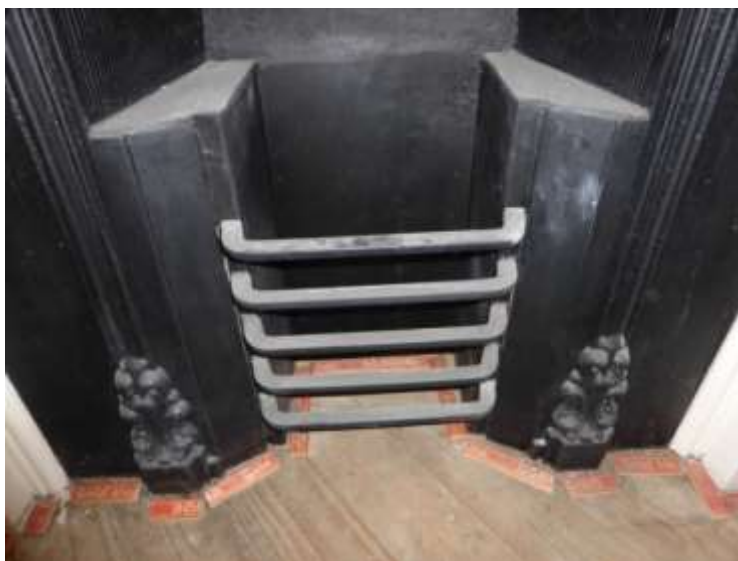
Figure 14: 20 th century floorboards running under the refurbished coal grate in F1
