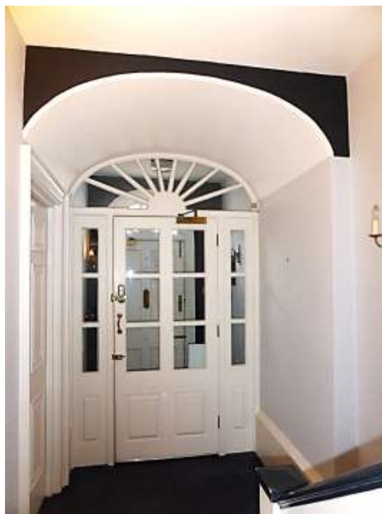
Figure 6: Lobby with 20 th century internal door and fanlight in G1
