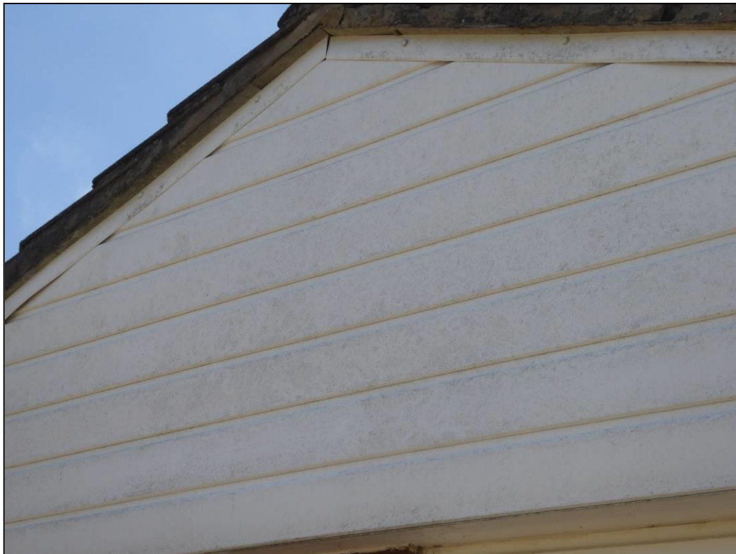
Figure 7. Example of uPVC cladding, 6 Courtenay Drive, Caversham. 26.07.18
