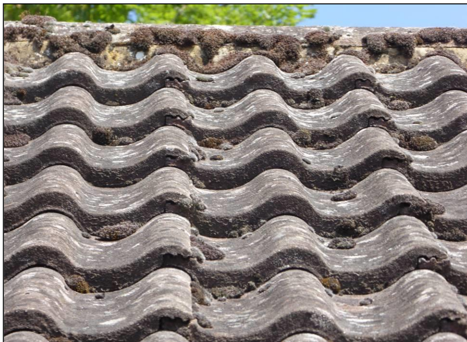
Figure 4. Example of roof tiles, 6 Courtenay Drive, Caversham. 26.07.18
