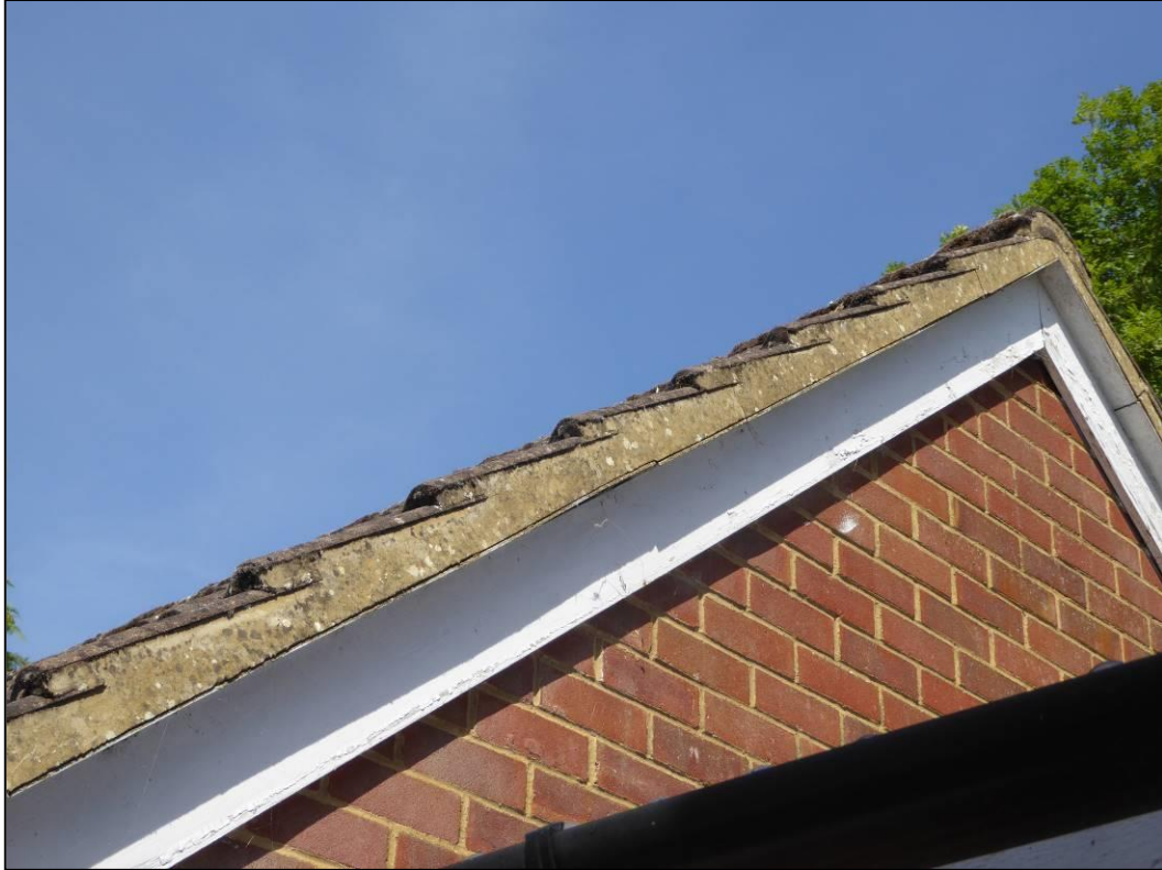
Figure 5. Example of verges, 6 Courtenay Drive, Caversham. 26.07.18
