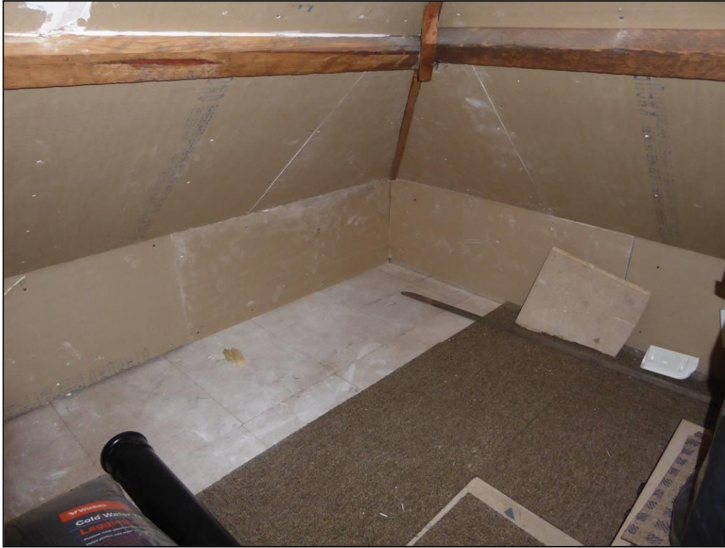
Figure 12. Loft space boarding and lining. 6 Courtenay Drive, Caversham. 26.07.18
