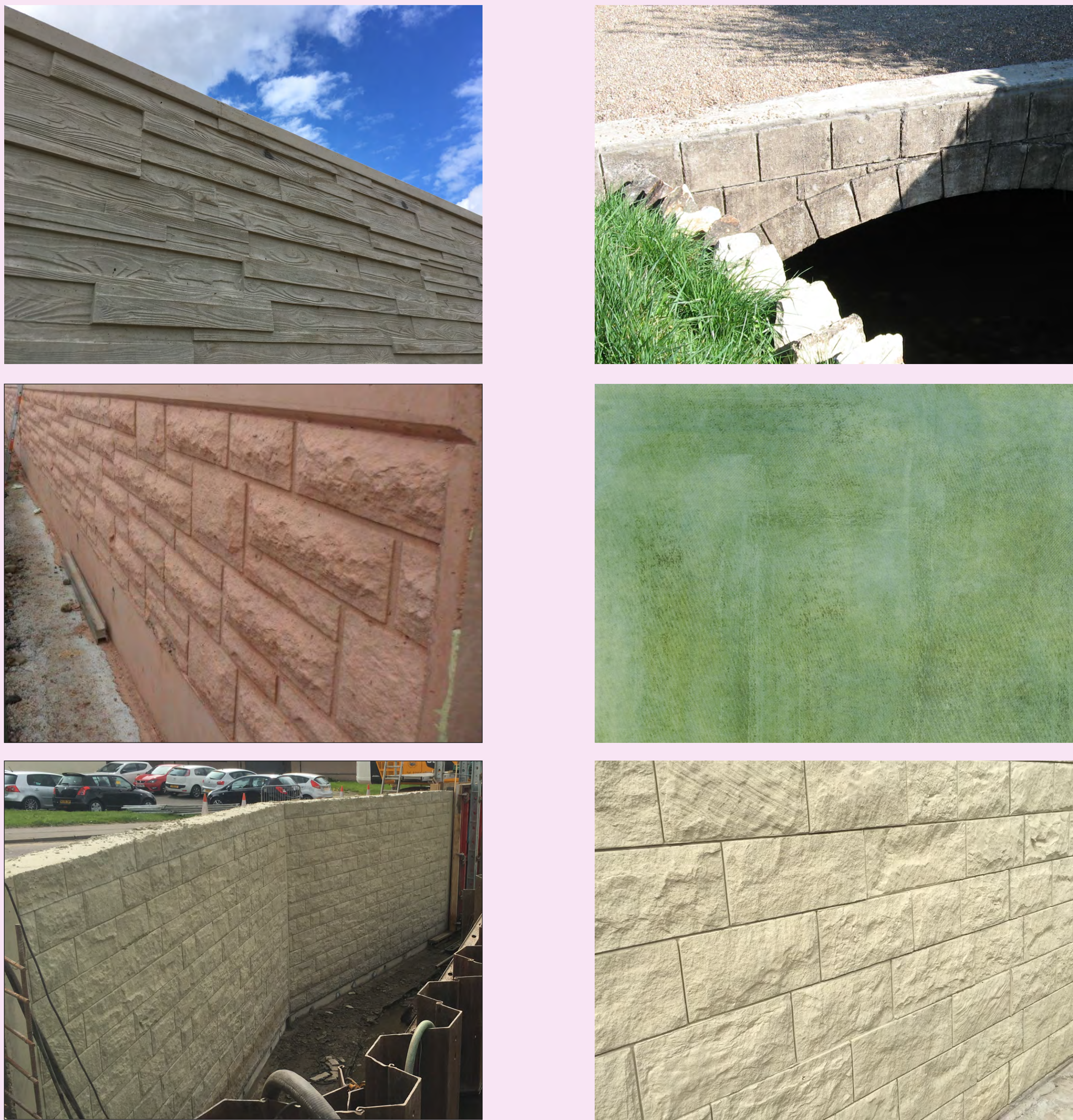
Example 3: Coloured pigment and/or textured concrete It is possible to pigment or texture the surface of the concrete.
