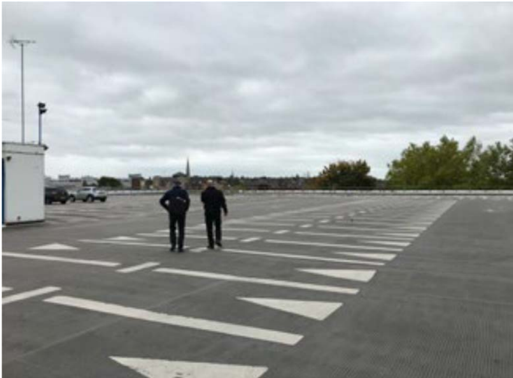
Figure 3 Second Storey Roof Car Park, above the Broad Street Mall
