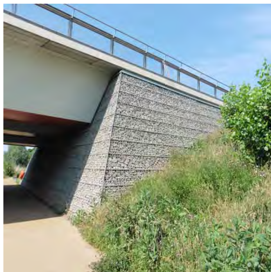
Figure 80. Example of a bridge abutment with gabion wall
