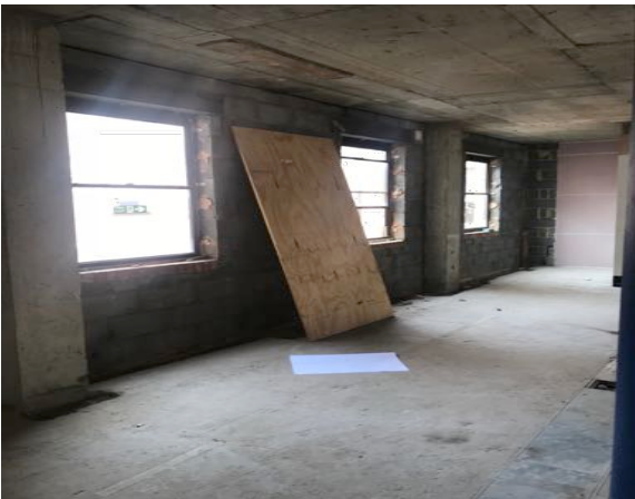
EXISTING REAR WALL TO LIGHTWELL DEMOLISHED TO ACCESS EXTENSION.
