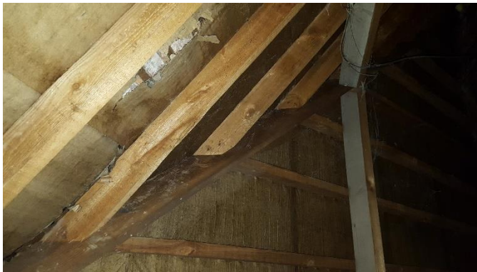
Internal – rip in felt roof space on western side of loft
