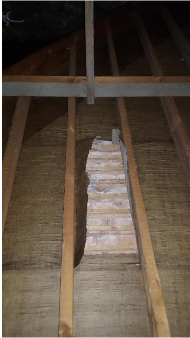
Internal – rip in felt roof space on western side of loft
