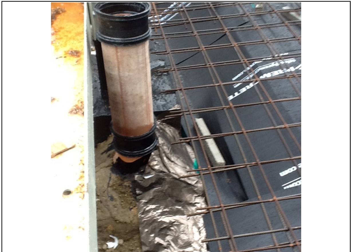
Overview pipe penetration detail
