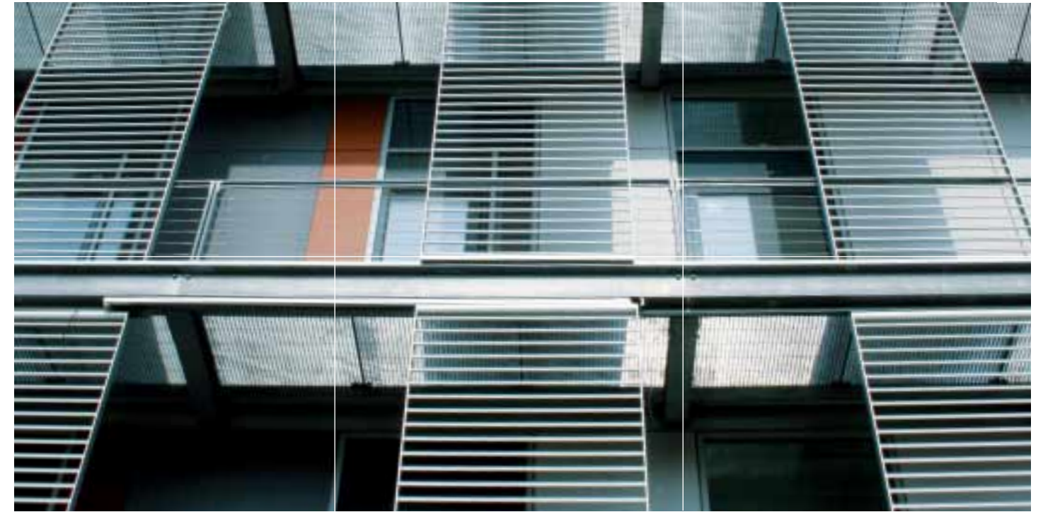
Folding shutters which automatically follow the sun's path.
