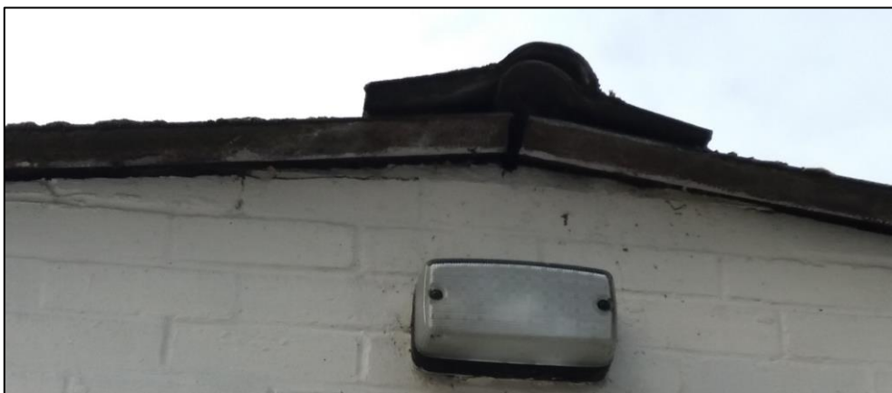
Figure 11 – showing open ended ridge fitting
