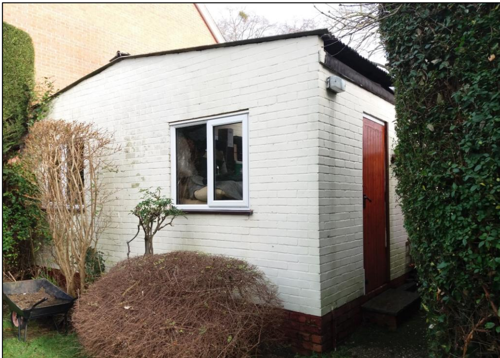
Figure 9 – rear of the garage showing corrugated roof and close-fitting timber boards at eaves
