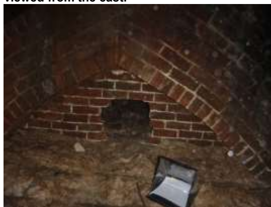
12. The main roof void showing the opening linking the two halves of the space.
