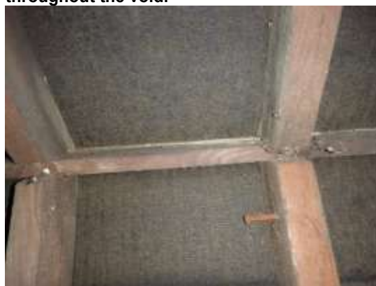
16. The intact bitumen felt lining the roof and lightly cobwebbed ridge.
