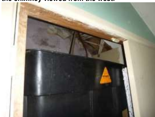
11. The enclosed cupboard containing the water tank; remainder of roof space converted to living space.
