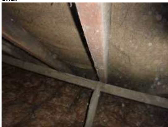
15. The eaves filled with fibre glass.
