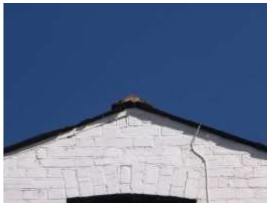
8. The slates fitted tightly to the brickwork at the south facing gable end.
