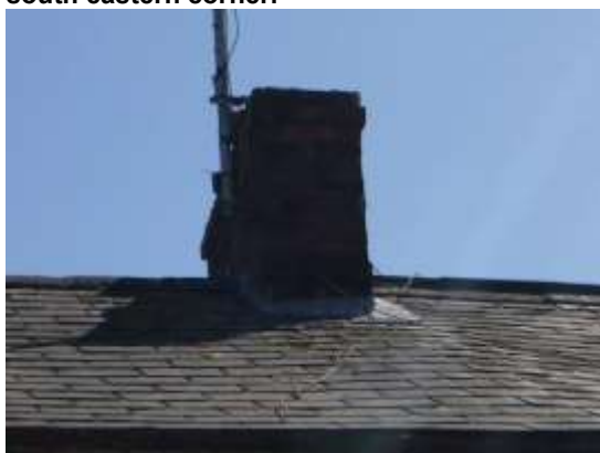
9. The flat slates and closely fitted lead around the chimney viewed from the west.
